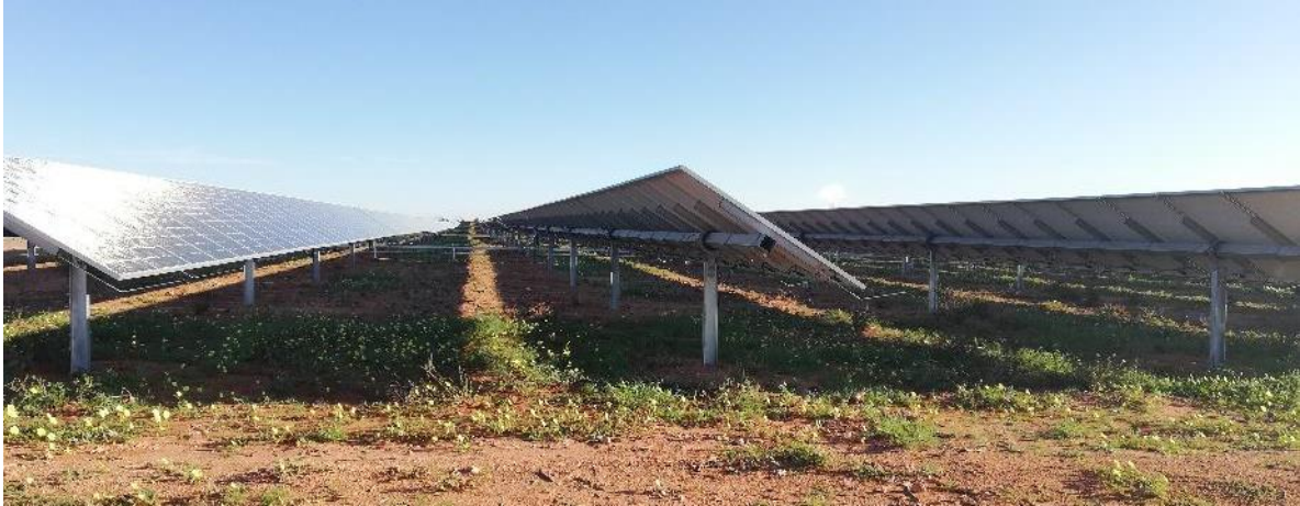
Single portrait module on a tracker (Photo – Cape EAPrac, 2019)
