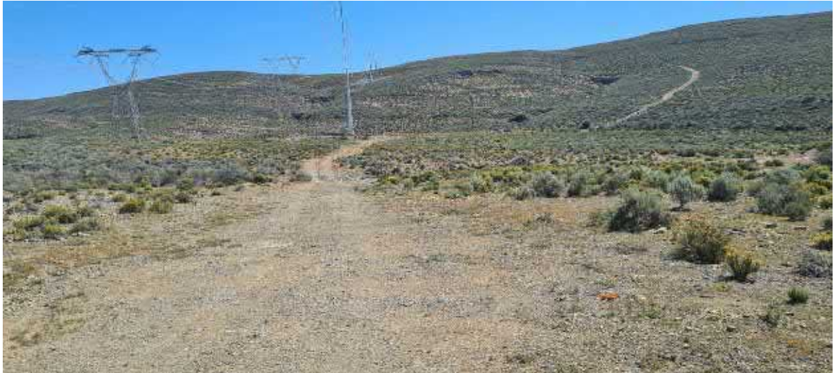
Figure 20: West of Substation
