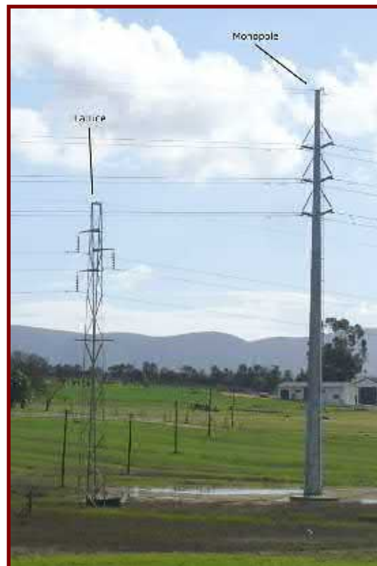
Figure 2: Conventional lattice powerline tower compared with a steel monopole structure
