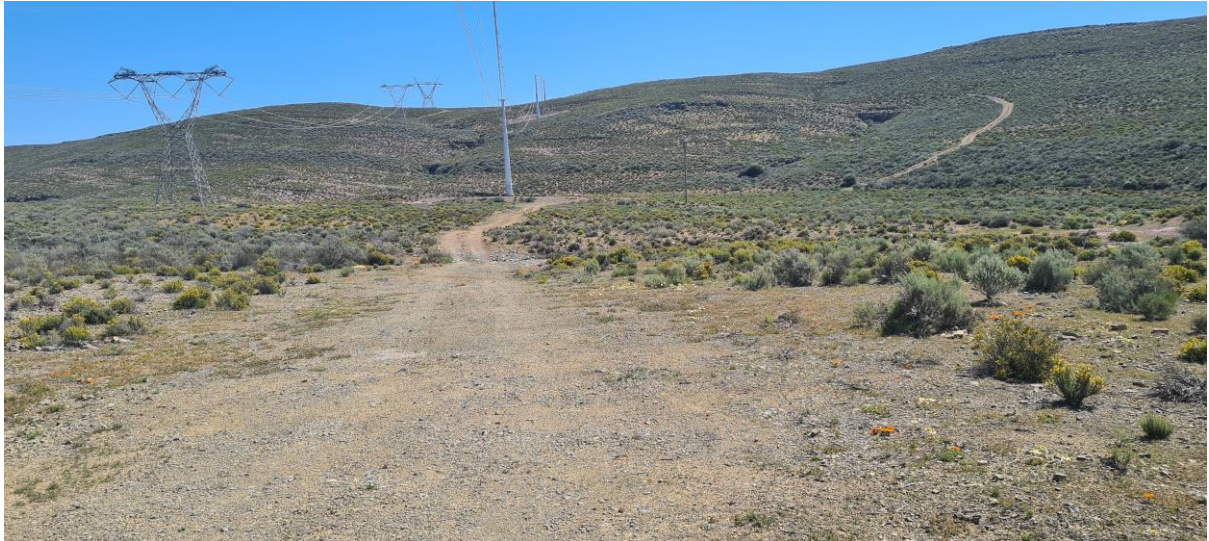
Figure 20: West of Substation
