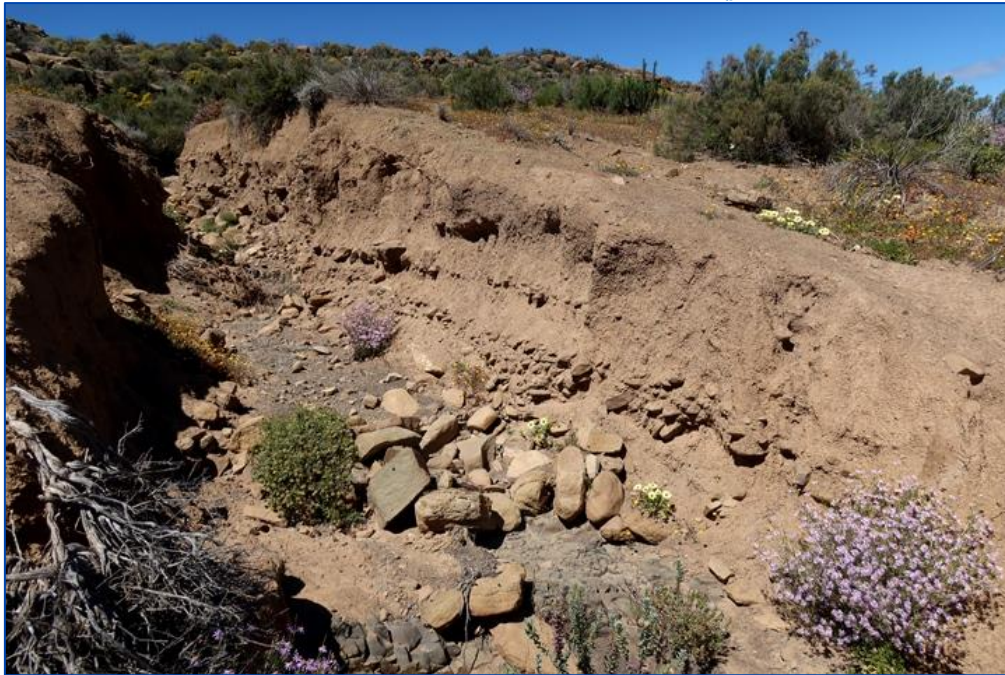
Figure 31: Thick, well-bedded apron of coarse gravelly to sandy colluvial deposits mantling the Abrahamskraal Formation bedrocks on the footslopes of Ruiter se Kop, Orange Fontein 203. These unconsolidated cover sediments are generally of low palaeosensitivity.
