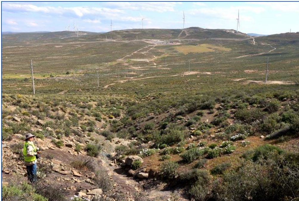
Figure 8: View southwards from Perdeplaas se Berg towards the new Karusa WEF substation on De Hoop 202. Grid Options 1A and 2A will traverse the low-relief terrain in the middle ground where bedrock exposure is very limited.
