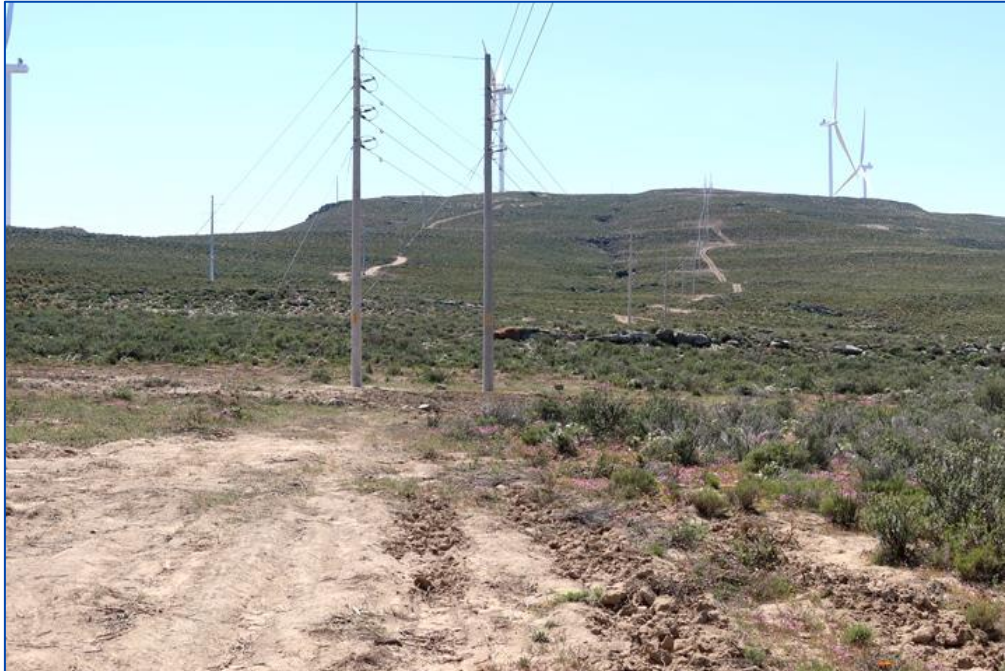
Figure 11: New powerline access routes running north from the Karusa WEF substation. Grid Options 1A and 2A would follow a similar corridor. Access roads in this area will mainly impact low palaeosensitivity superficial deposits.
