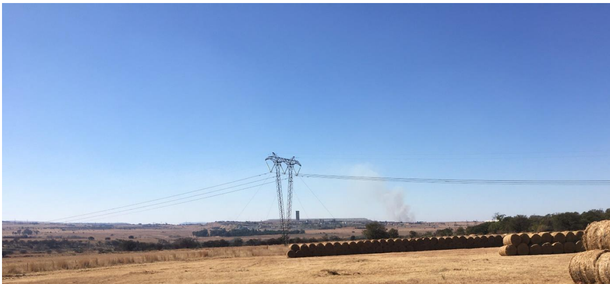
Figure 11: High voltage overhead powerline within the PAOI.
