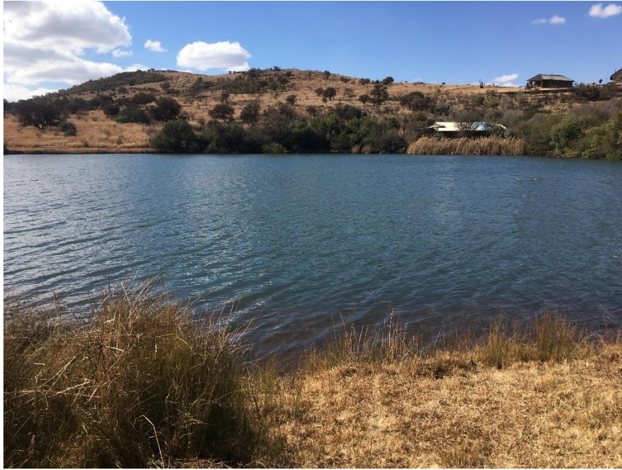
Figure 9: Large dam within the PAOI.
