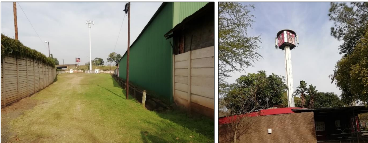
Plate 5: Communications infrastructure (reception towers) within the site.
