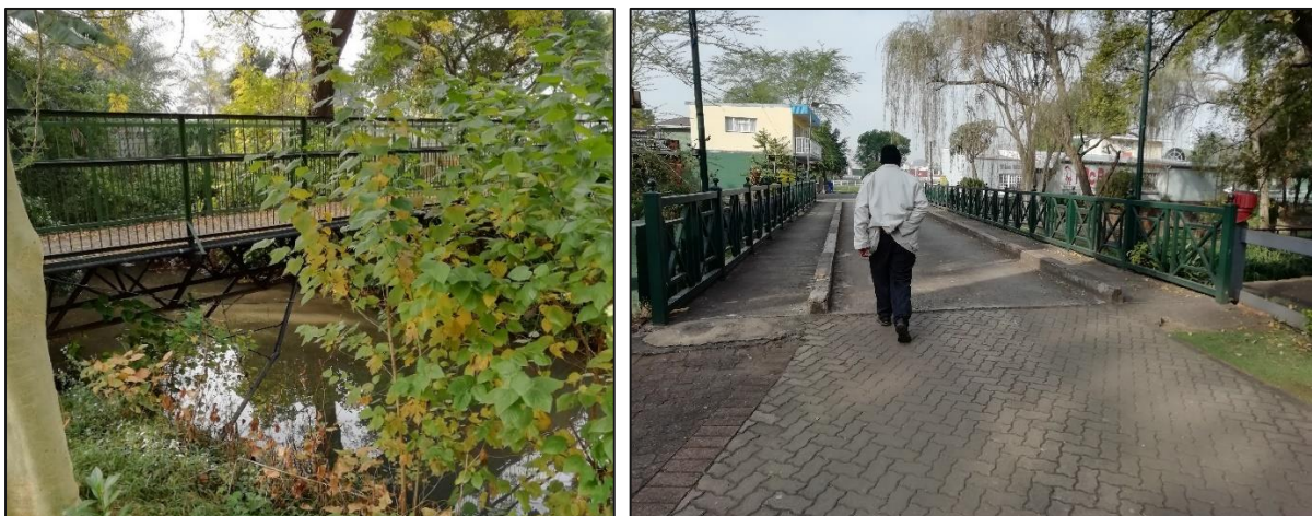
Plate 2: Examples of some of the bridges crossing the Dorpspruit River.
