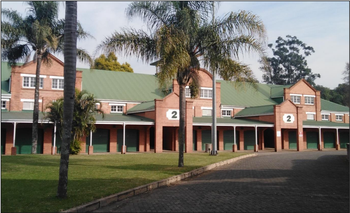
Plate 8: Industrial Hall which constitutes an important heritage building.
