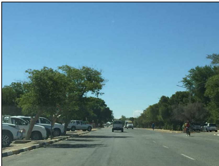
Photograph 1.4.12. Overview of the main road in the town of Kakamas.
