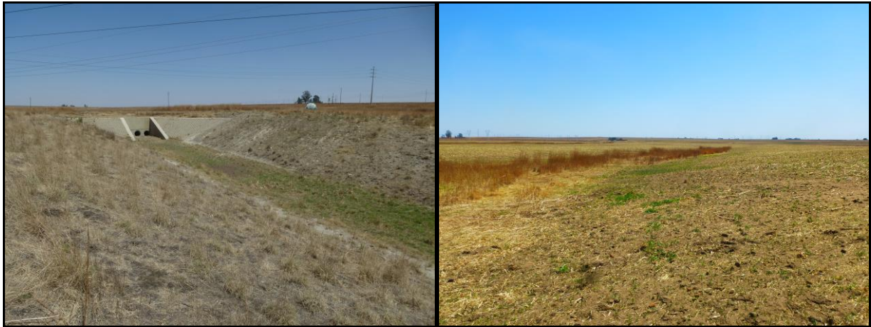
Figure 13. Photographs of the wetlands within the Block D area (clockwise from top left): Excavated channel and subsided area.
