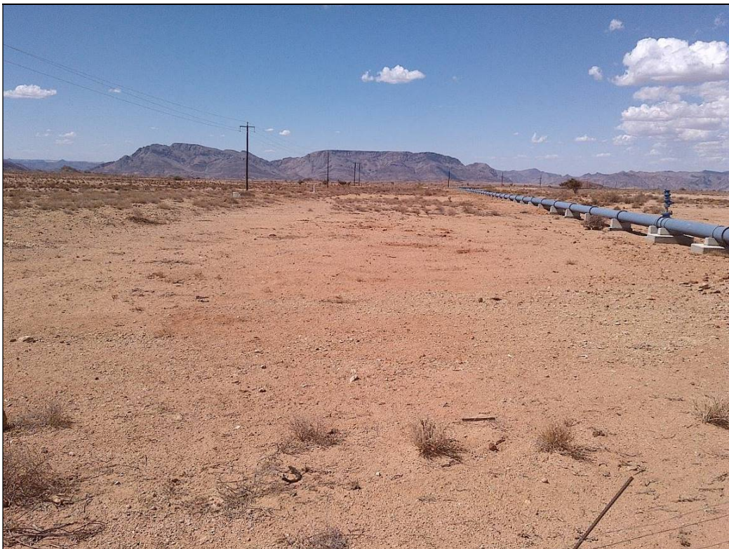
Figure 6. General site conditions- indicating high visibility and existing infrastructure.
