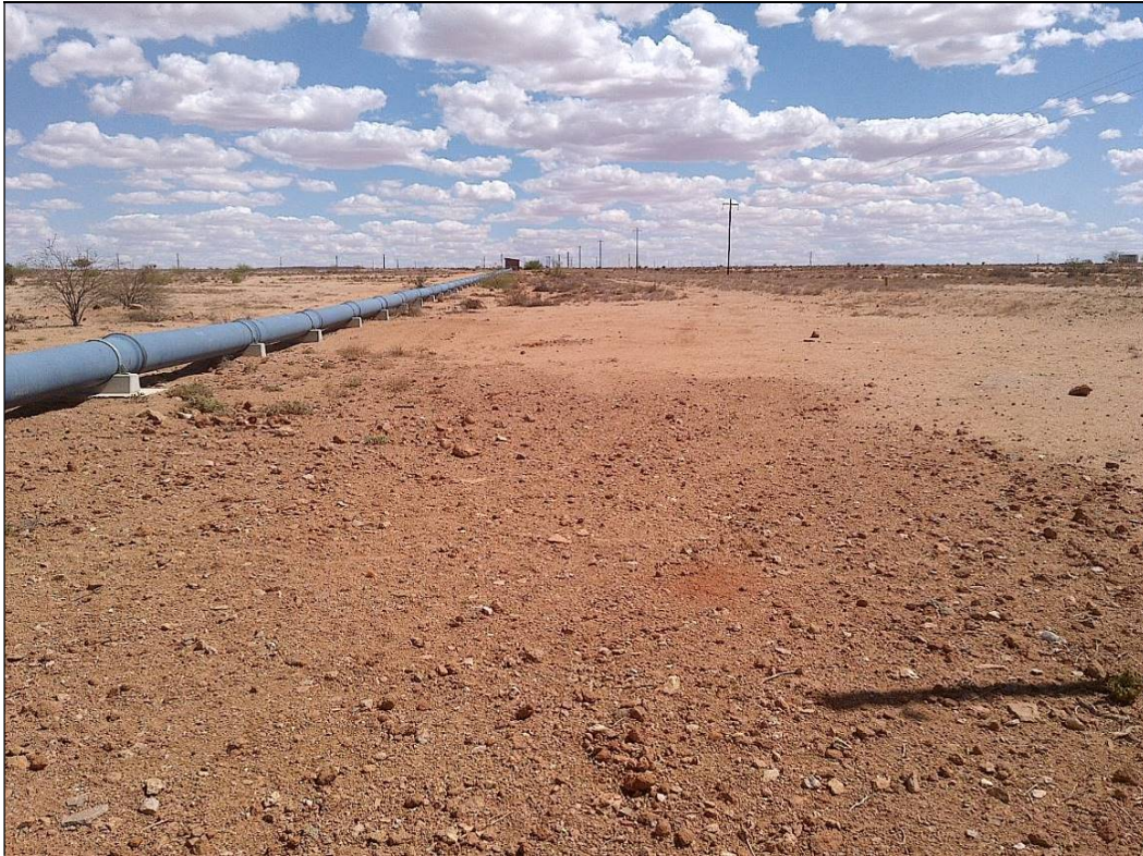
Figure 5. General site conditions- indicating high visibility and existing infrastructure.
