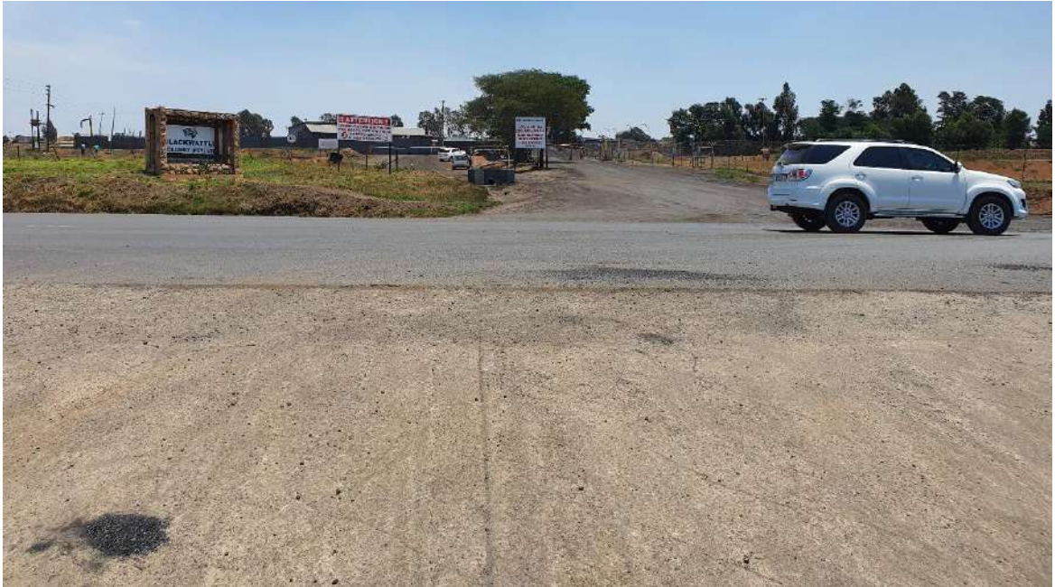
Photo 14: Looking west along the Access Road towards the R35 at the Colliery Access access road (note the small staggered layout)
