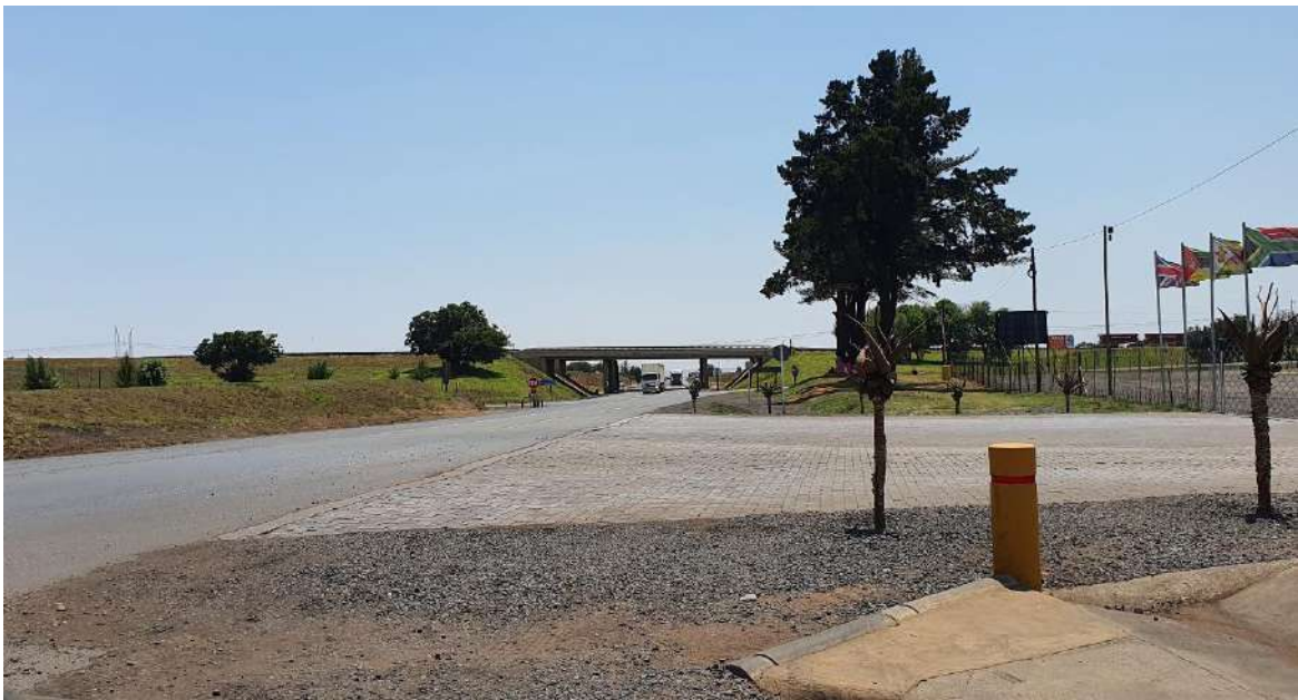
Photo 11: Looking north over the truck Stop access towards the N4 Interchange.
