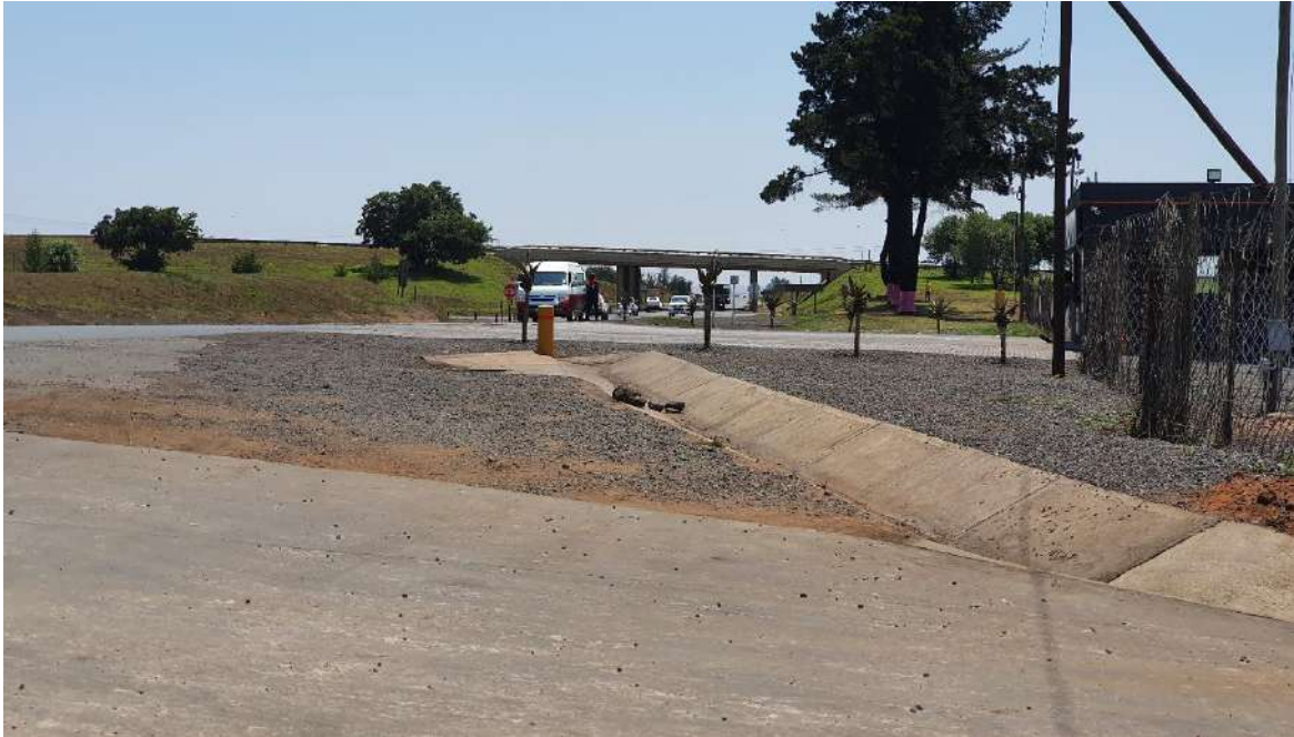
Photo 12: Looking north over the truck Stop access from the Access Road towards the N4 Interchange.
