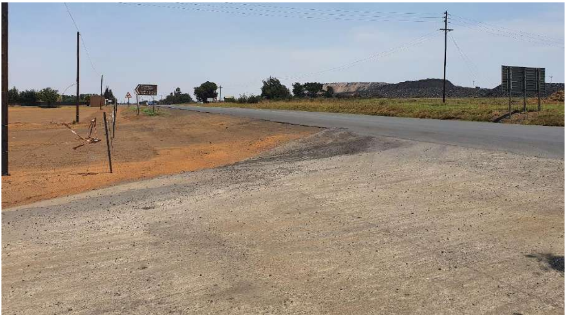
Photo 15: Looking south at the R35 from the Access Road
