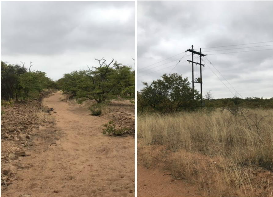
Figure 3-5 | Constructed drainage channel and overhead power line running inside and parallel to the Regina site boundary
