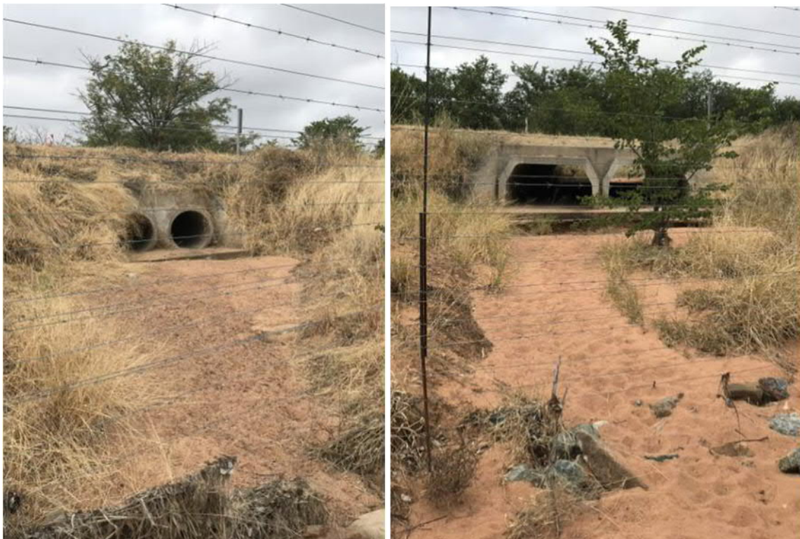
Figure 3-3 | View of culverts on the Drumsheigh portion on the southern boundary
