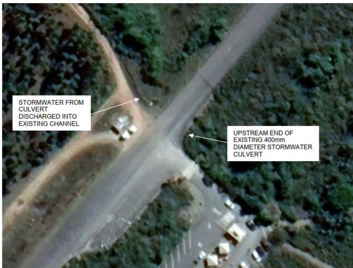
Figure 4-8: Existing stormwater infrastructure
