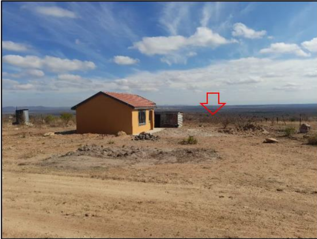
Figure 39: View from the Sekuruwe settlement directly south of the proposed Sekuruwe WTW.
