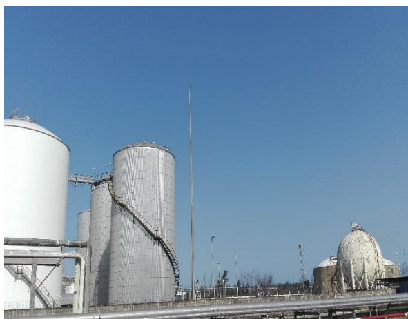
Figure 10: An existing mast next to Bidvest tanks
