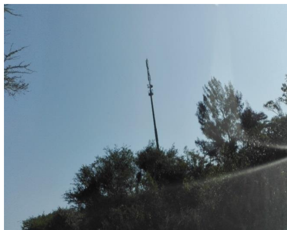
Figure 11: Existing Tall structures within RBCT
