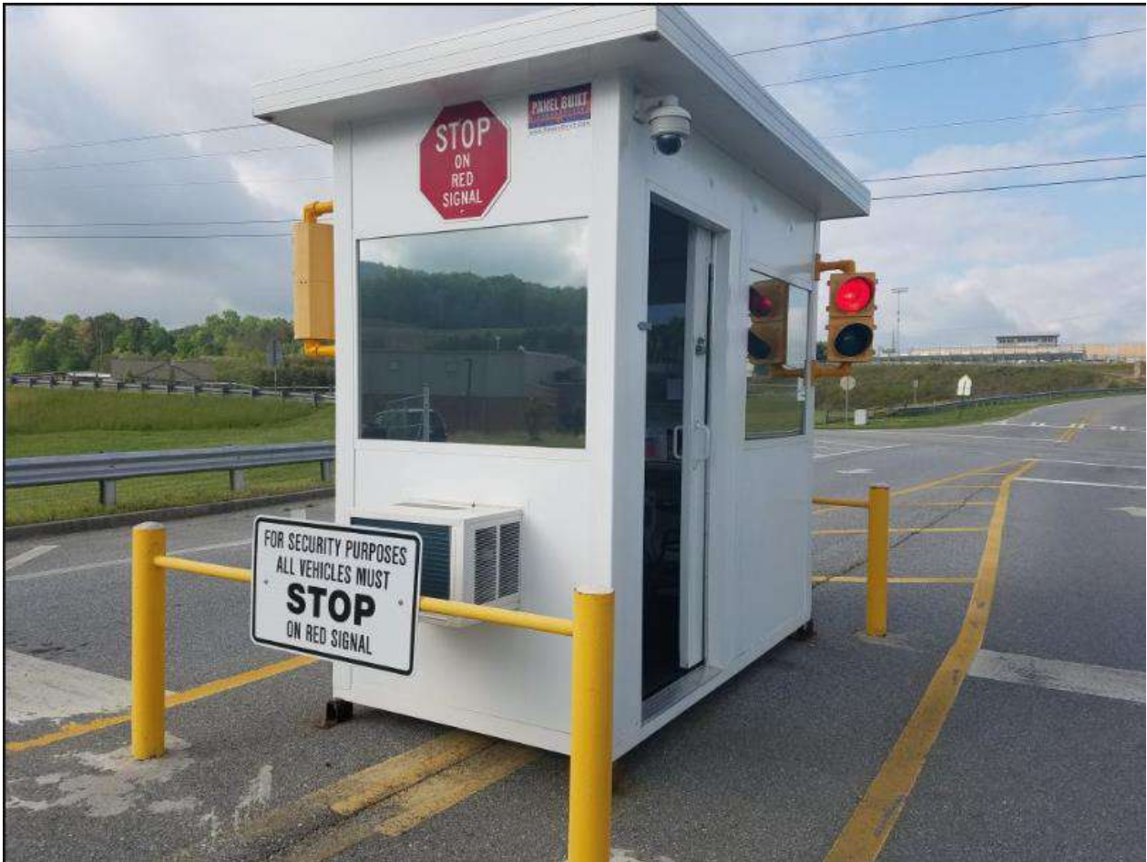
Image 6: Typical example of a guard house
