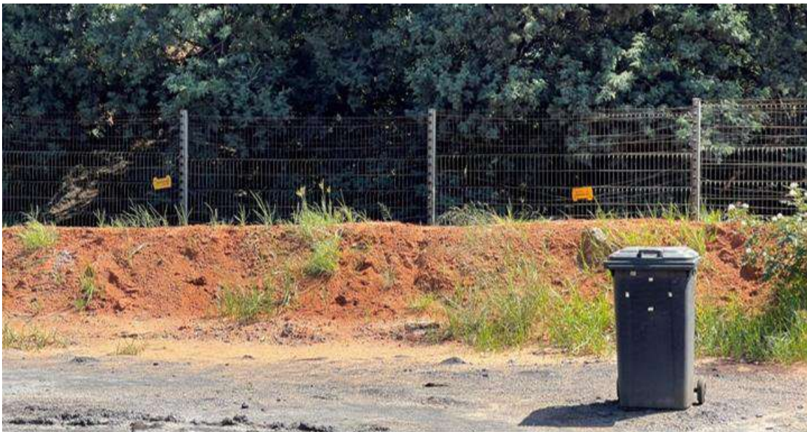
Image 5: Clearvu as the typical Fencing that will be used on site. (Synman, 1998)
