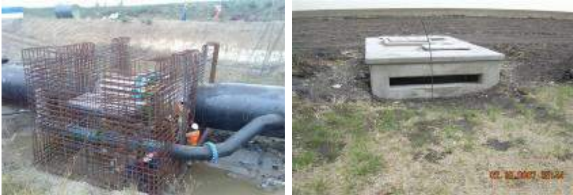
Figure 92: Typical examples of chambers (left - during construction; right – completed)
