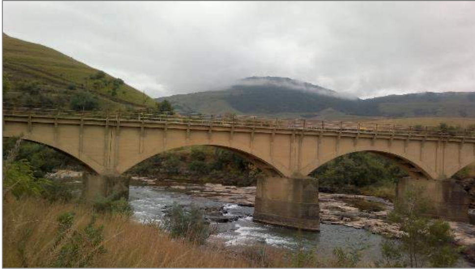
Figure 184: Deepdale Bridge (Jean & Prins, 2015)
