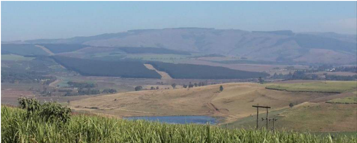
Figure 172: South-western view of timber plantation (in background) traversed by raw water pipeline routes to WTW Options 1 and 3
