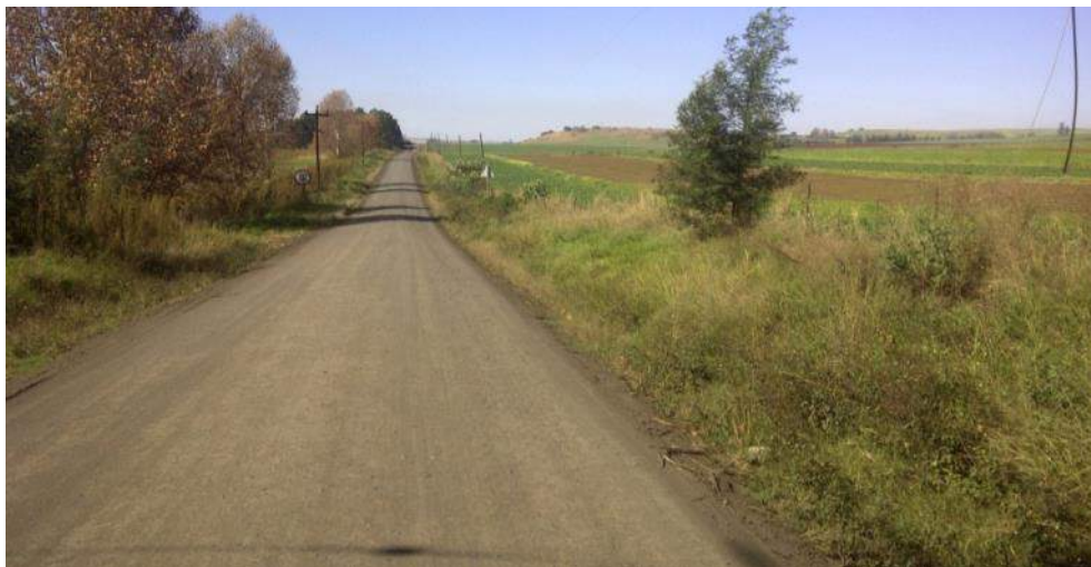
Figure 68: South-easterly view - raw water pipeline to WTW Option 3 (along D360)
