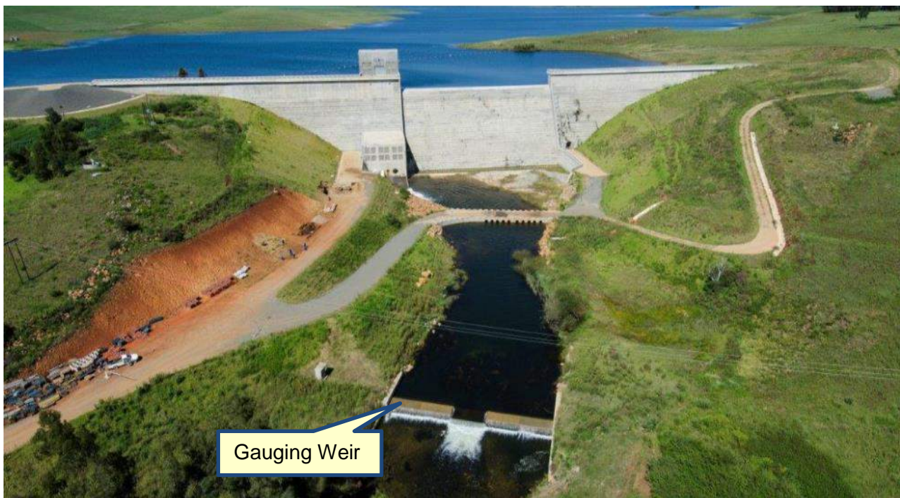
Figure 51: Example of a gauging weir downstream of Spring Grove Dam
