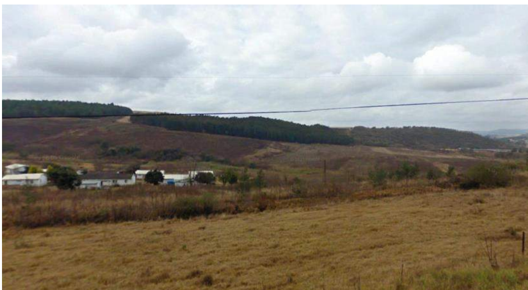
Figure 66: South-easterly view - raw water pipeline to WTW Option 2 (P334 crossing)
