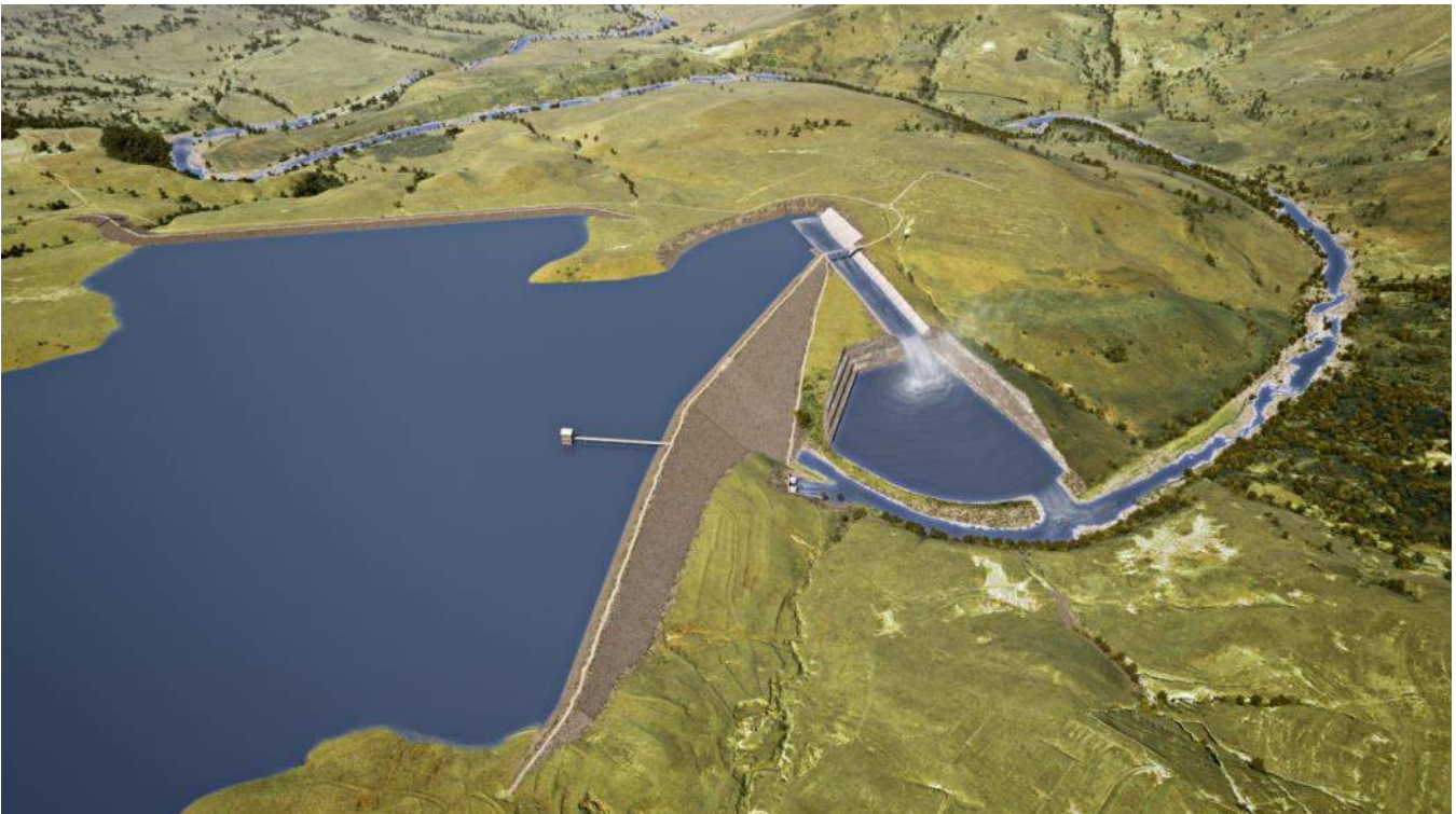
Figure 31: Three-dimensional layout of Smithfield Dam (view 2)
