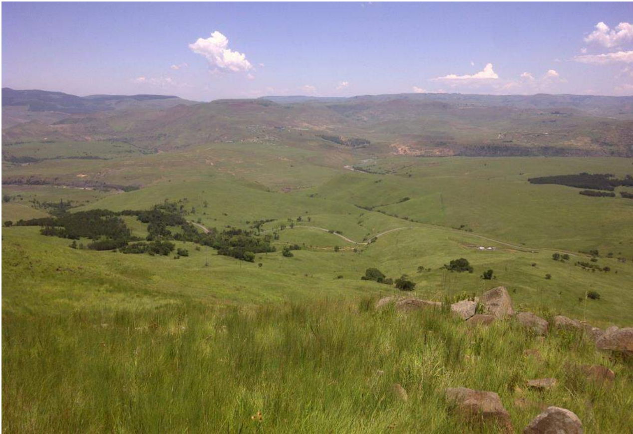
Figure 210: View of Smithfield Dam site
