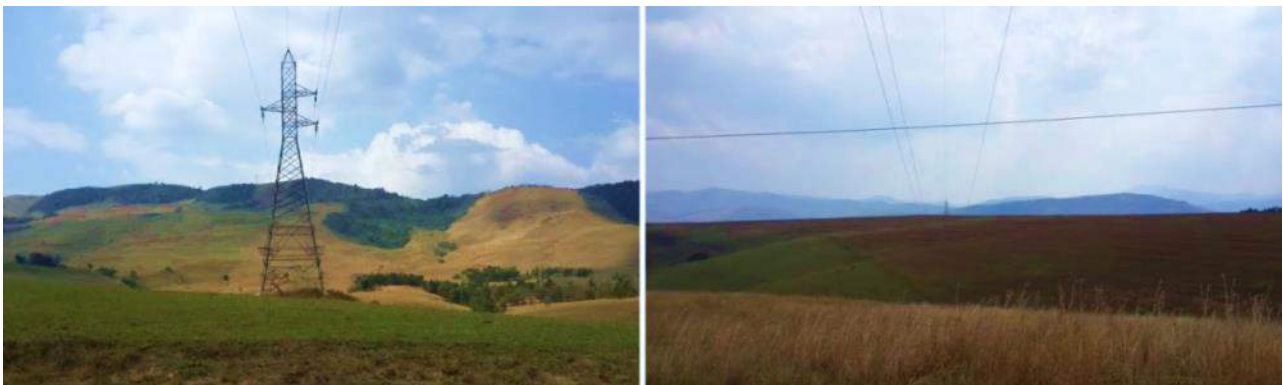
Figure 78: Transmission line at Smithfield Dam site to be deviated
