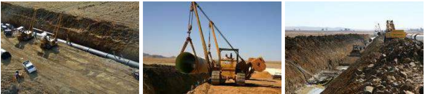
Figure 91: Typical trench excavation and pipe installation activities
