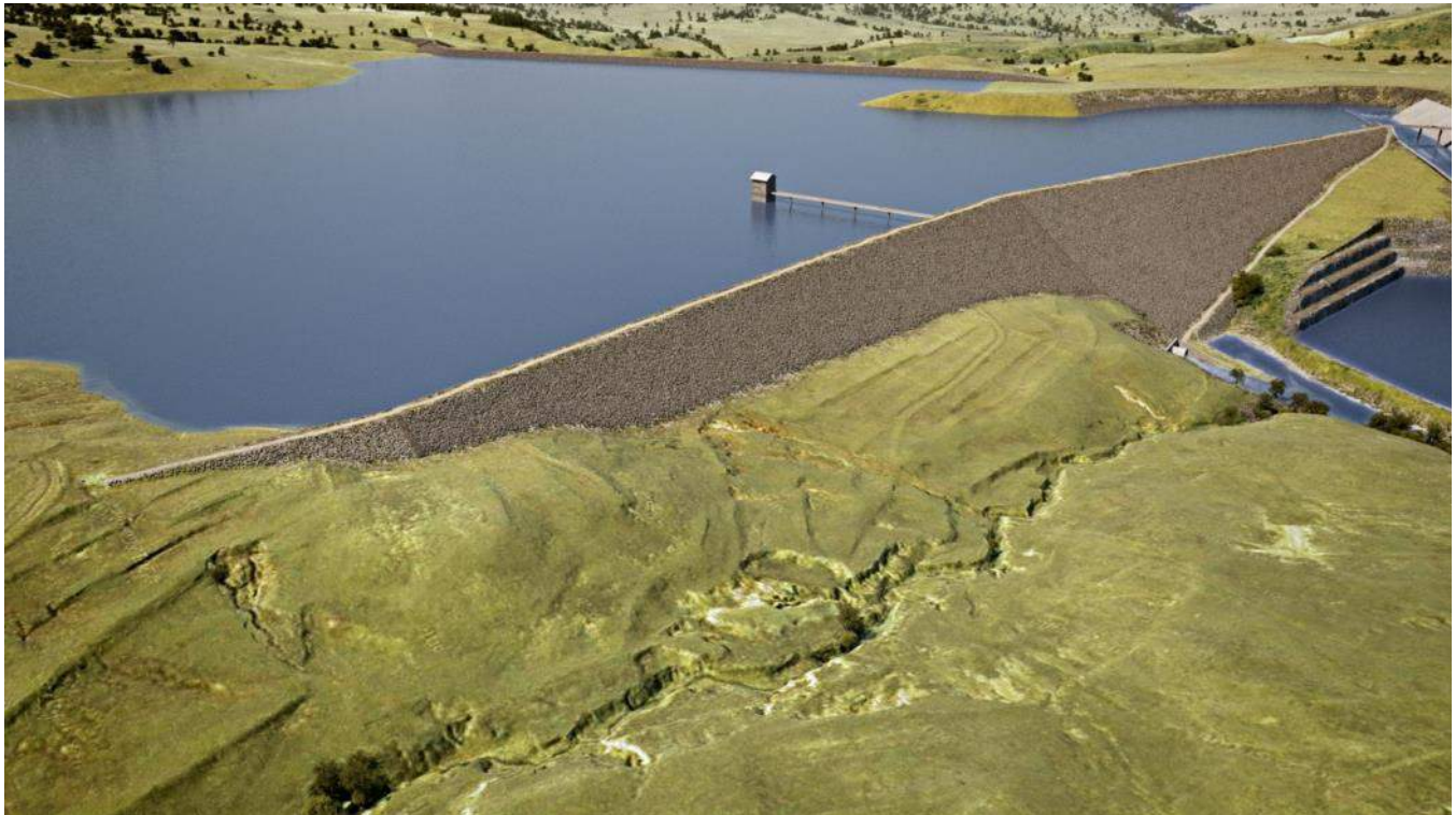
Figure 32: Three-dimensional layout of Smithfield Dam (view 3)
