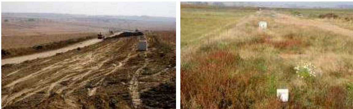
Figure 93: Typical views of reinstated (left) and rehabilitated (right) pipeline routes
