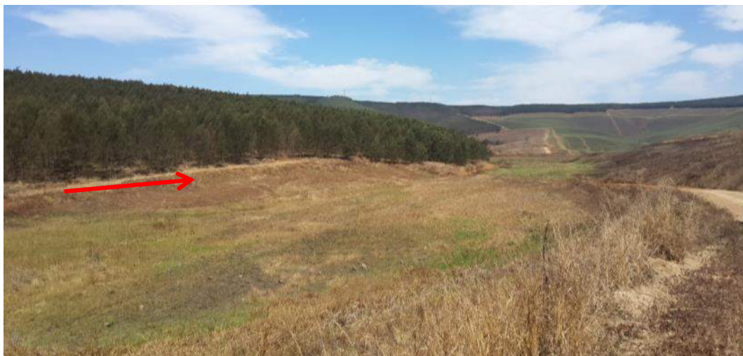
Figure 71: Southern view - raw water pipeline to balancing dam
