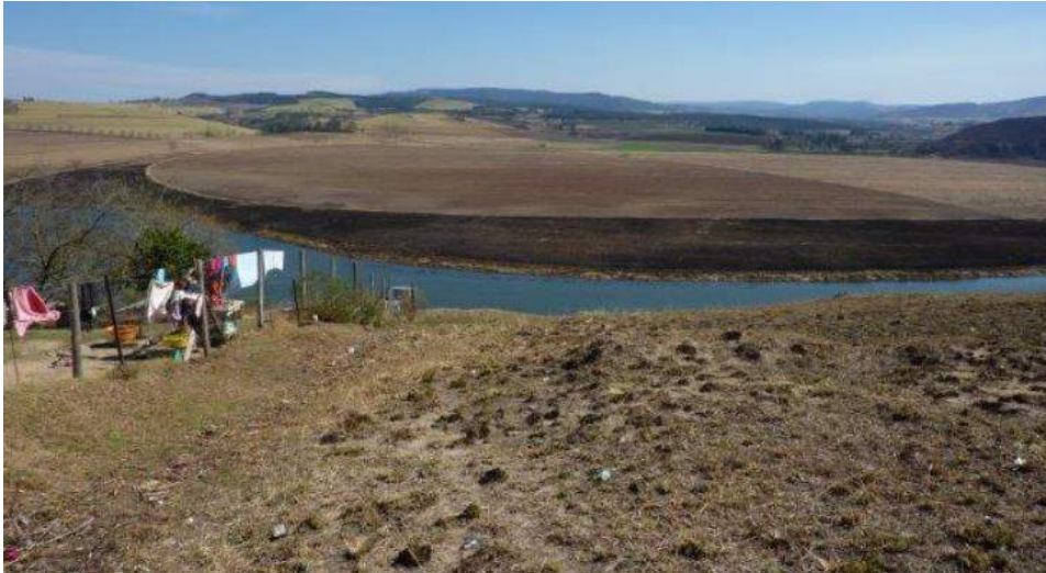
Figure 41: Western view along Option 1 pipeline route (Mapstone Dam crossing)
