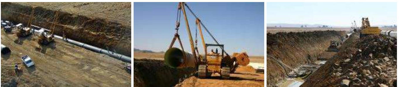
Figure 76: Typical trench excavation and pipe installation activities
