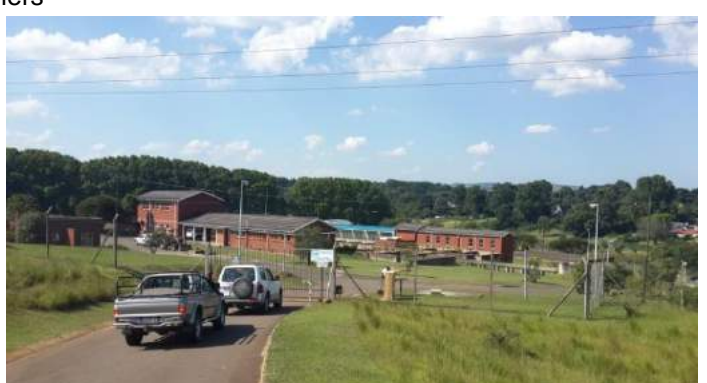
Sludge treatment plant
