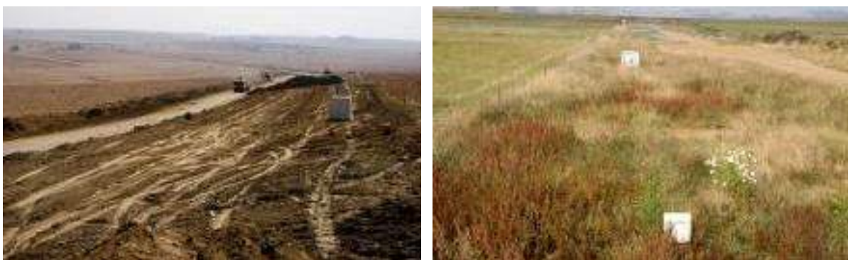
Figure 78: Typical views of reinstated (left) and rehabilitated (right) pipeline routes
