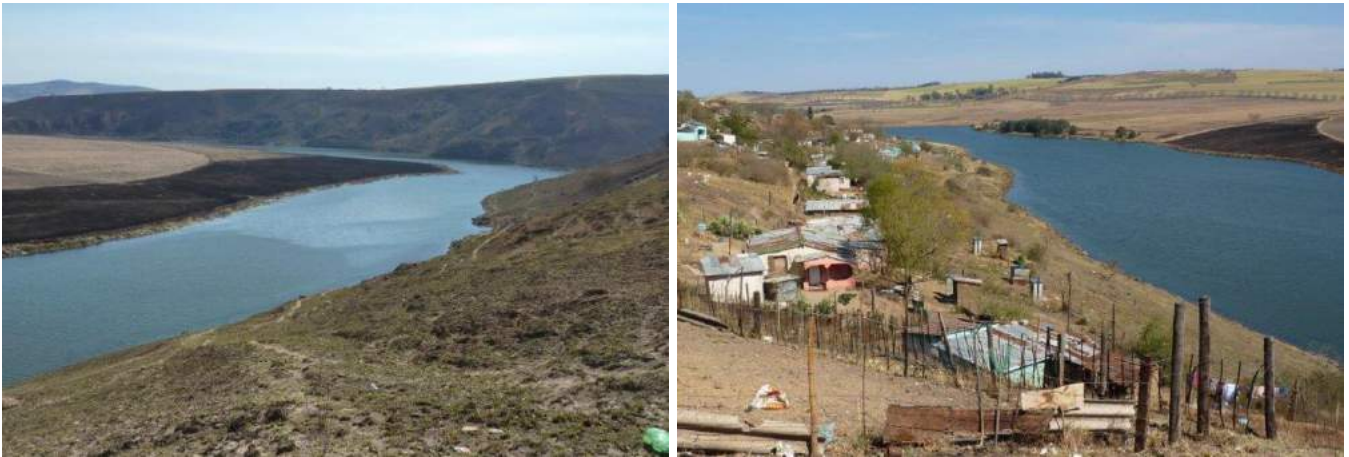
Figure 99: North-west (left) and south-west (right) view of Mapstone Dam near proposed crossing of pipeline route Option 1
