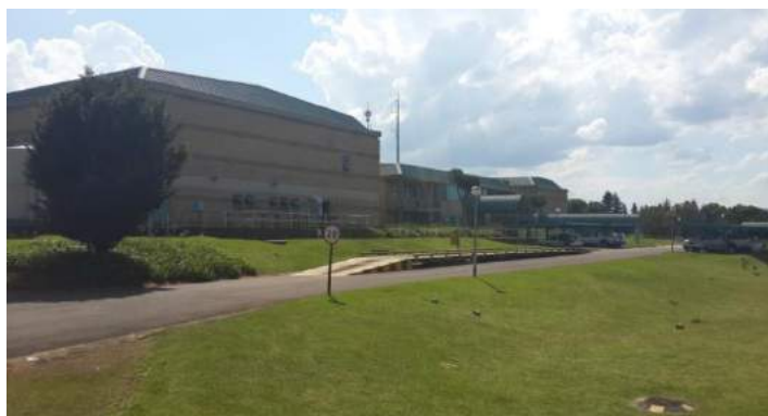
Offices and plant
