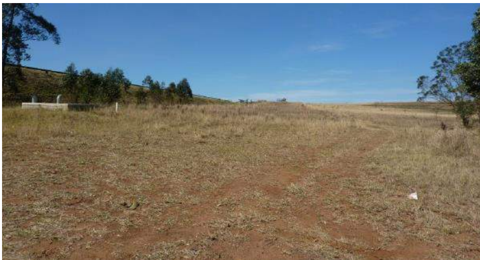
Figure 45: Tie-in to '57 Pipeline
