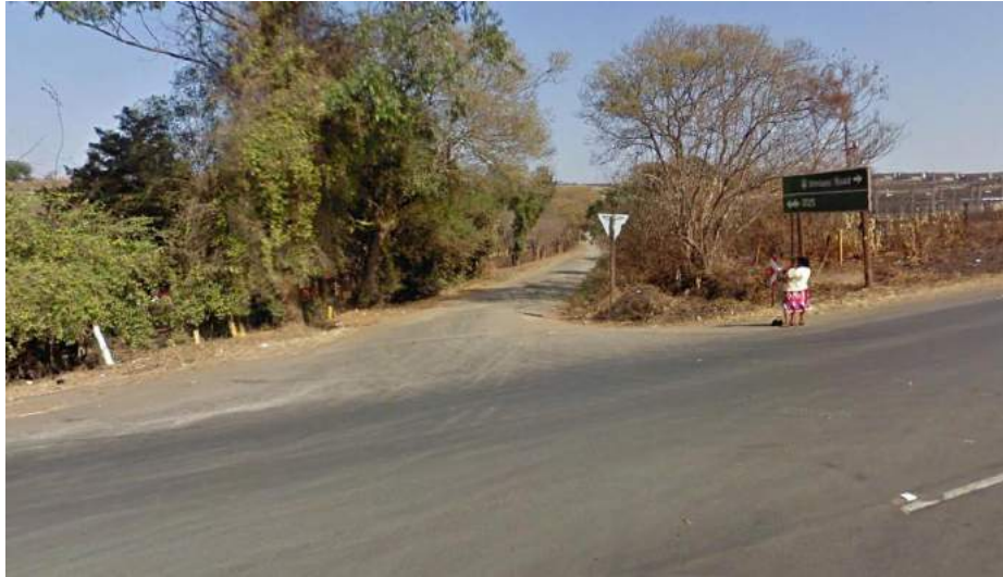
Figure 43: Westerly view along Option 1 pipeline route next to D125 (R603 crossing)
