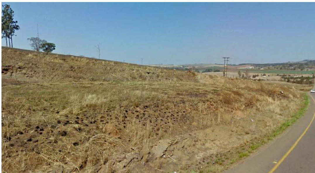
Figure 58: South-easterly view along pipeline link to WTW 2 (R56 crossing)
