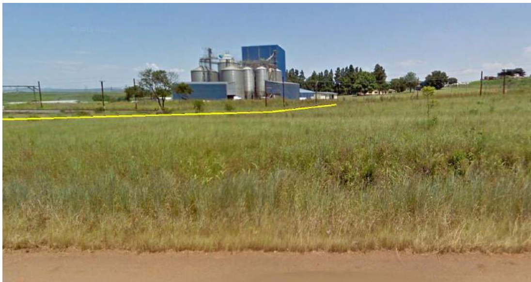
Figure 54: South-westerly view along Option 1D and Option 1E pipeline routes (yellow line) - railway crossing
