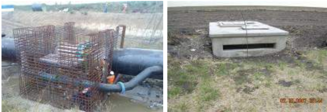
Figure 77: Typical examples of chambers (left - during construction; right – completed)
