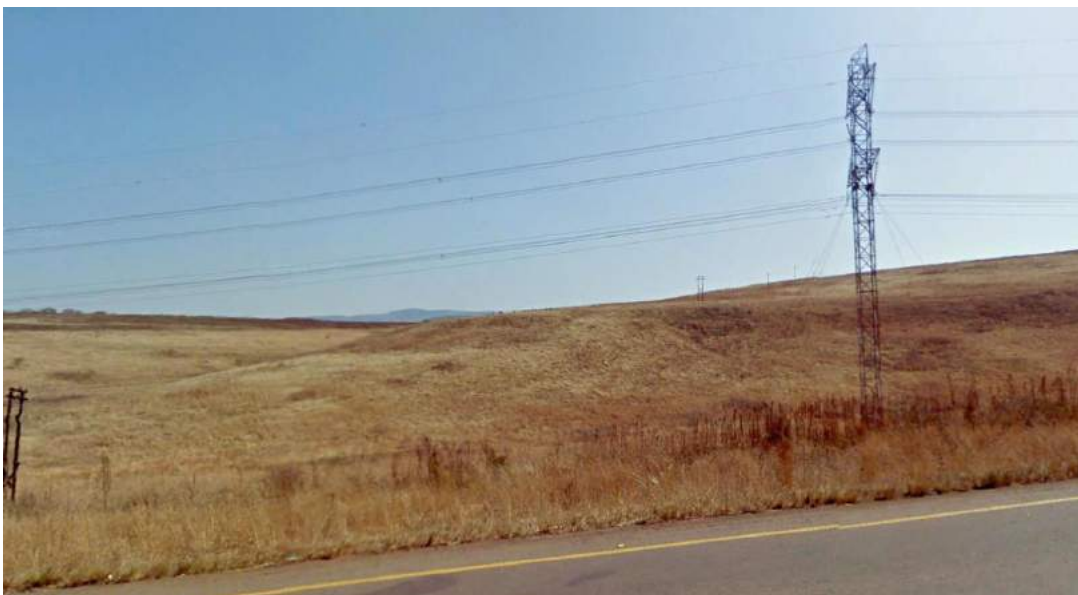
Figure 57: North-westerly view along pipeline link to WTW 2 (R56 crossing)
