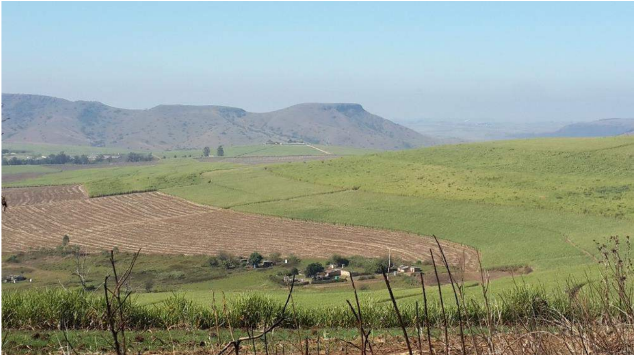
Figure 60: General view of WTW 3 site
