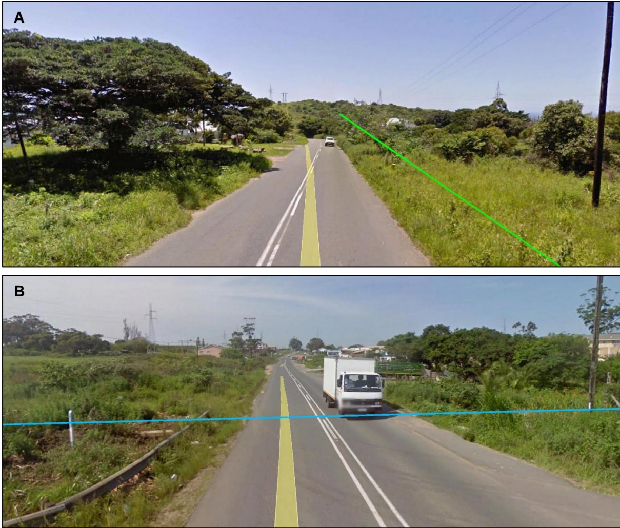
Figure 66: The roads traversed by (A) the gravity main from WTP 1 and (B) the gravity main from WTP 2 to the Quarry Reservoir
