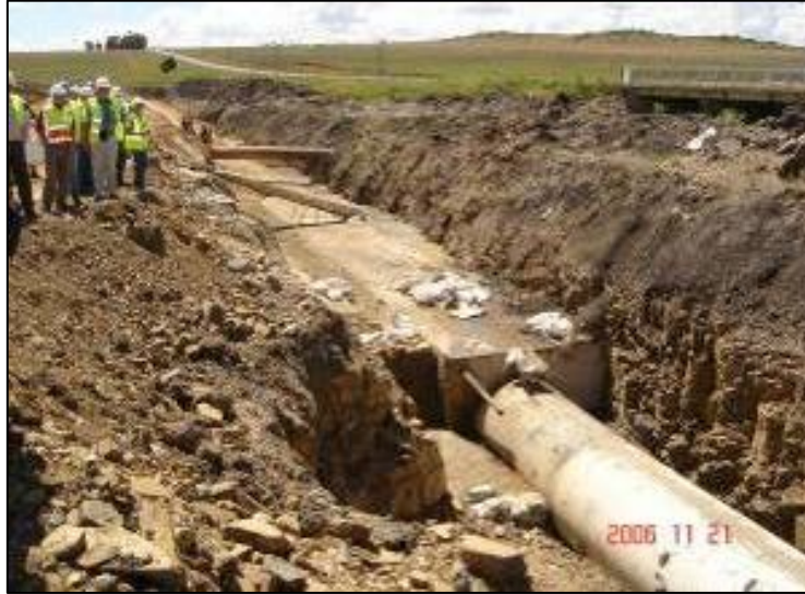
Figure 23: Typical river crossing showing concrete encased pipe section
