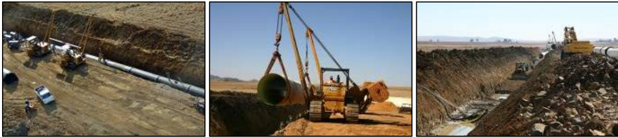
Figure 20: Typical trench excavation and pipe installation activities
