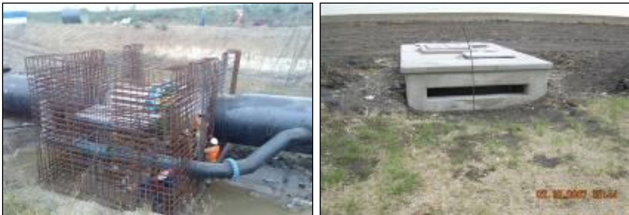
Figure 21: Typical examples of chambers (left - during construction; right – completed)
