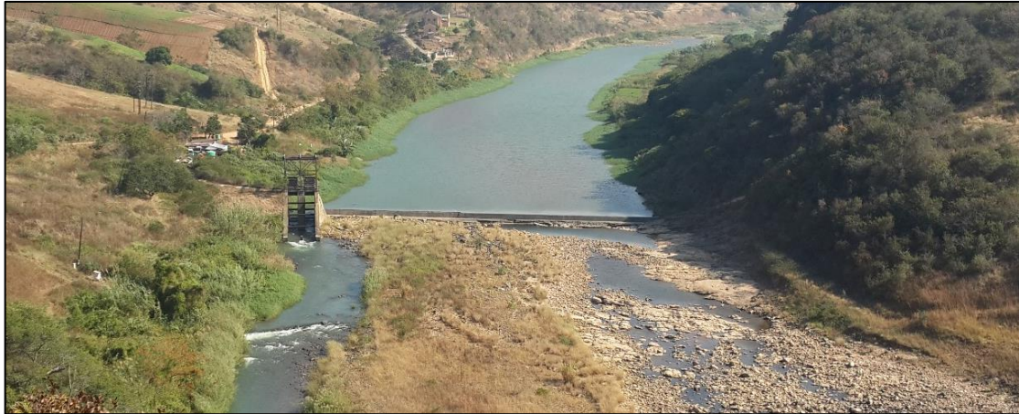
Figure 7: The existing Goodenough weir
