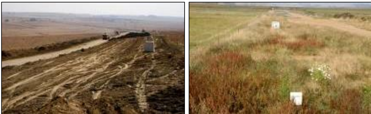
Figure 24: Typical views of reinstated (left) and rehabilitated (right) pipeline routes
