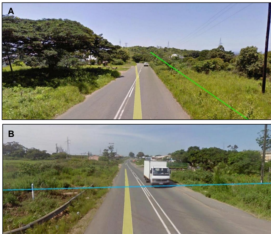
Figure 69: The roads traversed by (A) the gravity main from WTP 1 and (B) the gravity main from WTP 2 to the Quarry Reservoir
