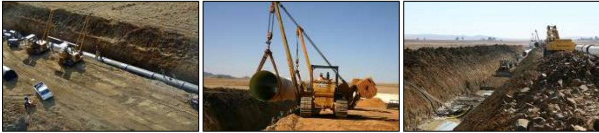
Figure 22: Typical trench excavation and pipe installation activities
