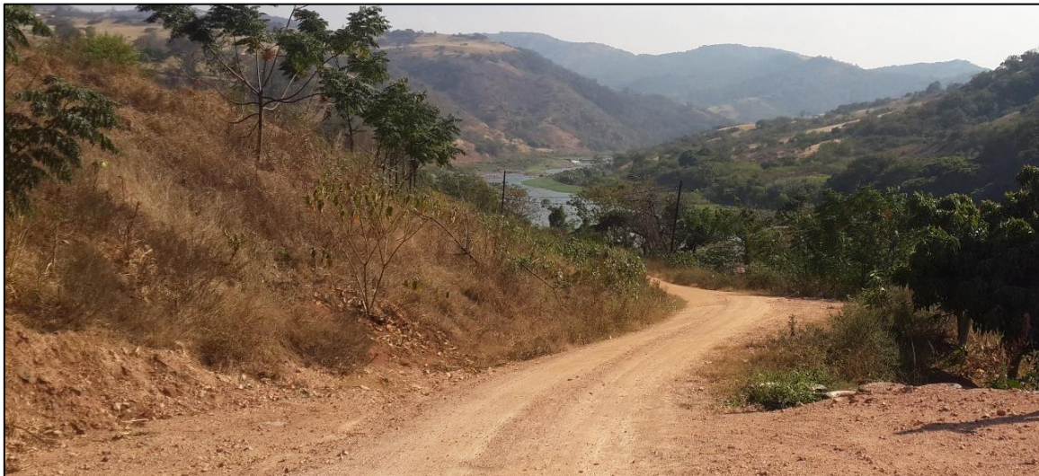
Figure 67: Dirt road near the existing Goodenough weir site
