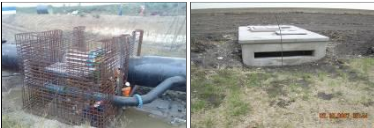
Figure 23: Typical examples of chambers (left - during construction; right – completed)
