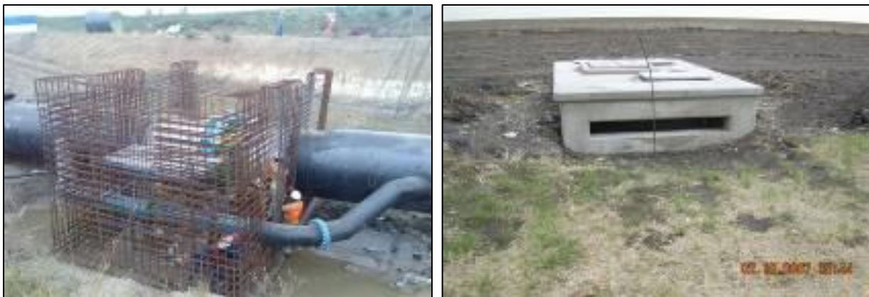
Figure 14: Typical examples of chambers (left - during construction; right – completed)
