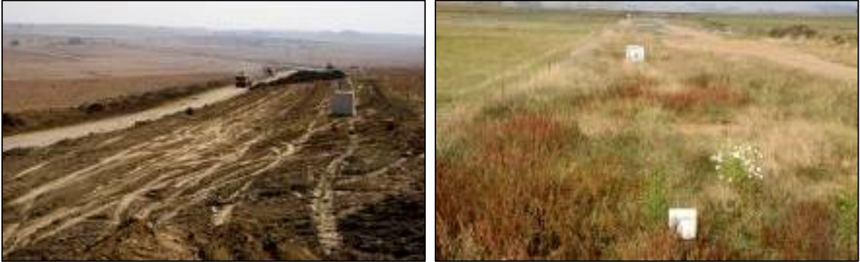
Figure 15: Typical views of reinstated (left) and rehabilitated (right) pipeline routes
