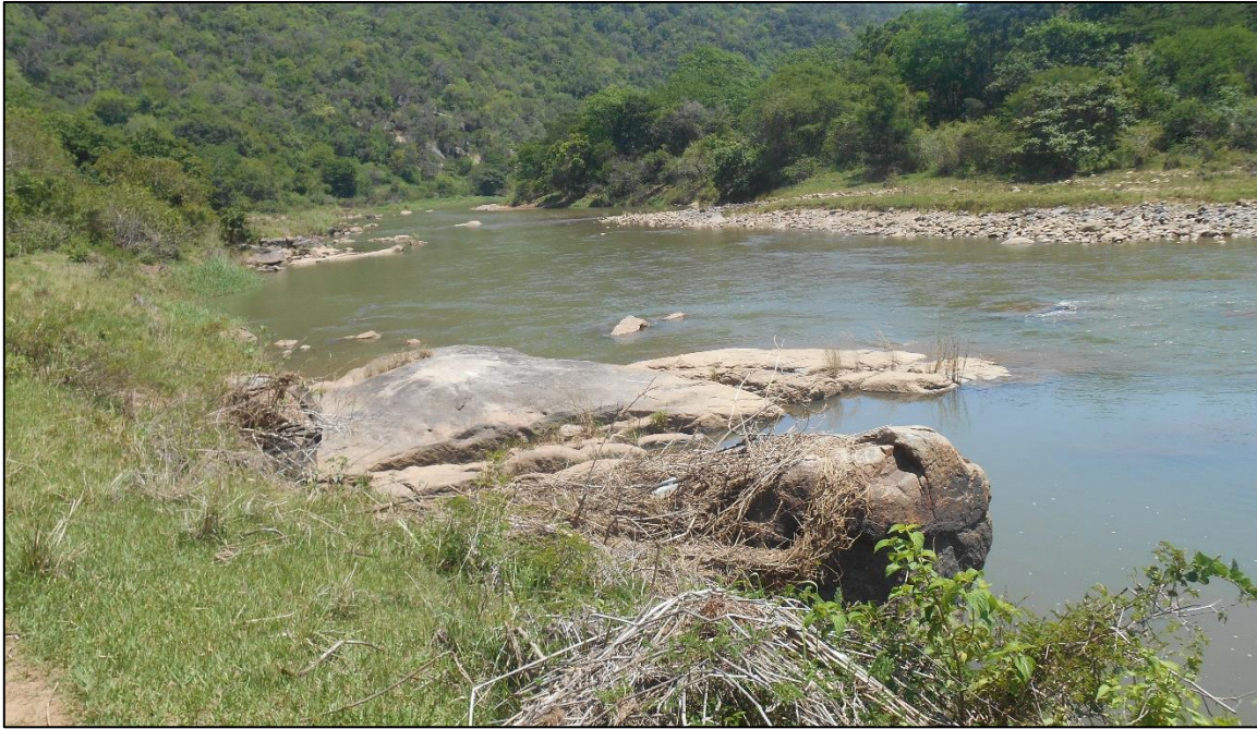
Figure 26: Ngwadini weir and abstraction works site
