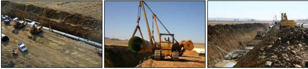
Figure 13: Typical trench excavation and pipe installation activities
