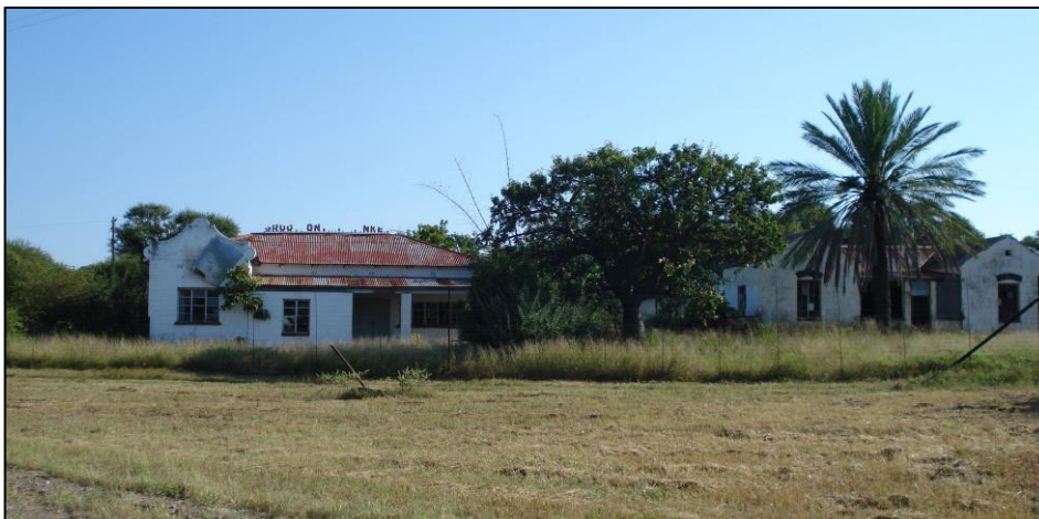
Figure 28: Example of an old structure in the study area
