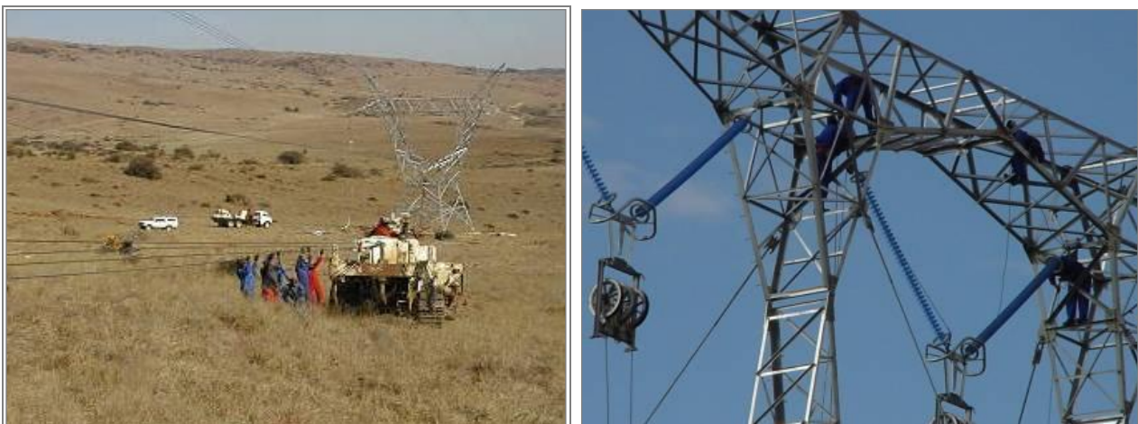
Figure 30: Stringing with pilot tractor (top) and pulleys (bottom)
