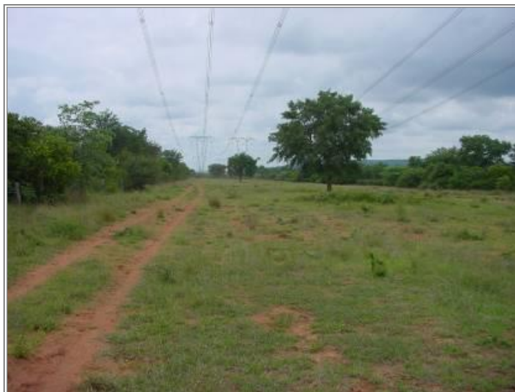
Figure 31: Example of an access road used for maintenance
