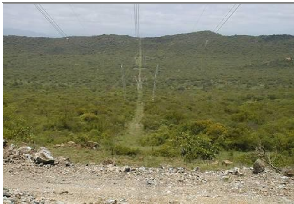
Figure 21: Vegetation clearance for stringing
