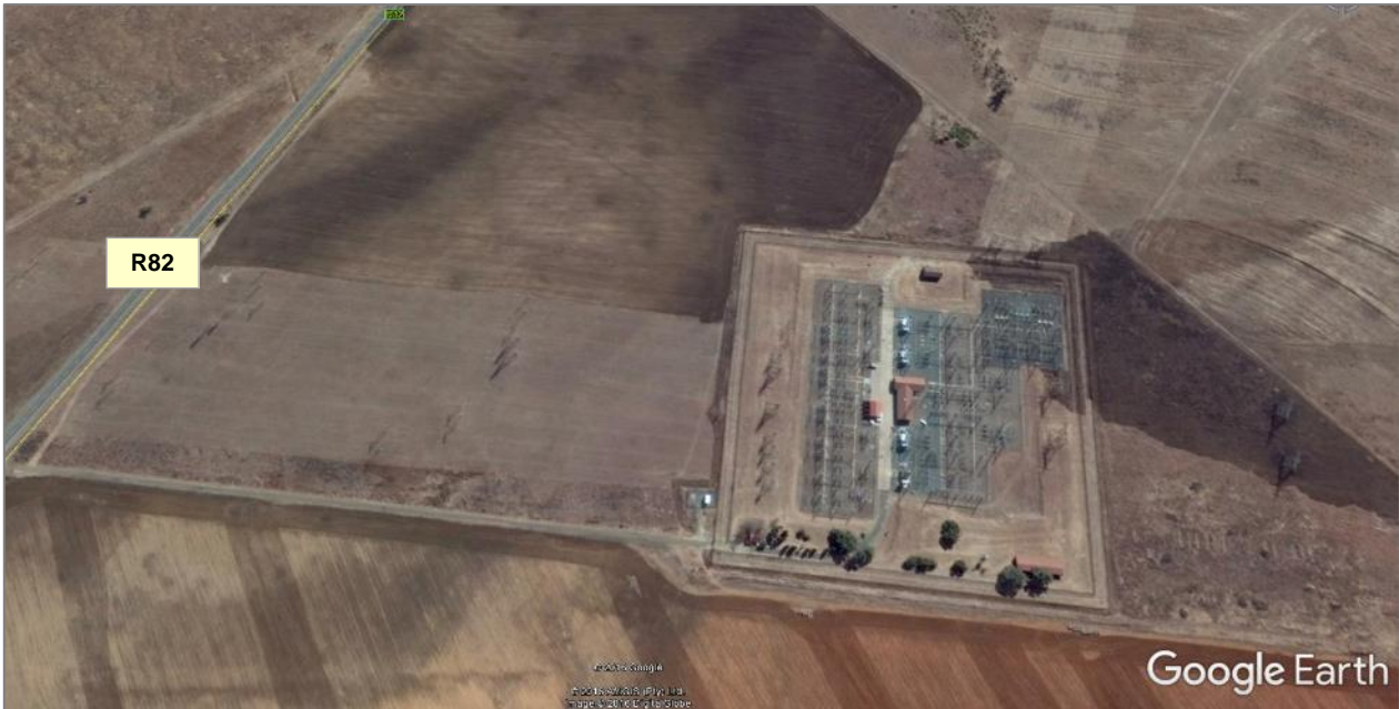
Figure 8: Makalu substation (Google Earth image)
