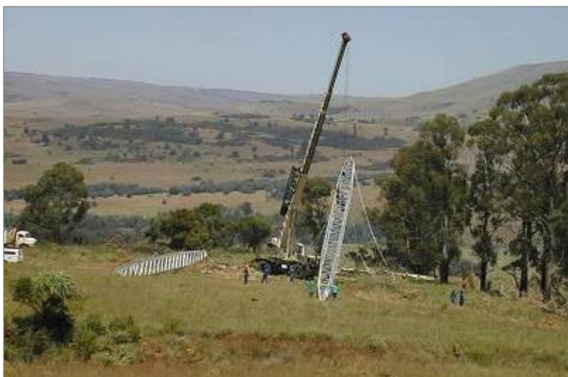
Figure 28: Erection of towers
