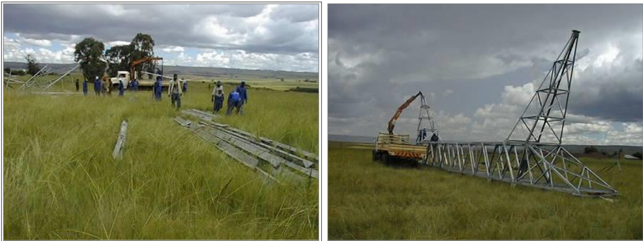
Figure 27: Delivery of steel (top) and assembly of tower (bottom)
