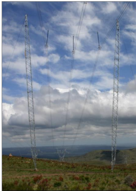
Figure 16: Tower Type 438 A - Cross Rope Suspension tower
