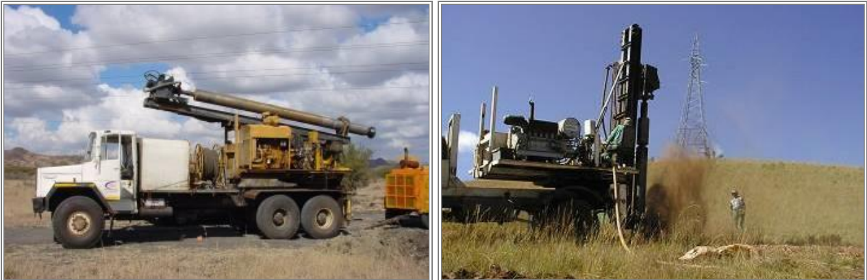
Figure 25: Drilling rig and generator (top) and excavation activities (bottom)
