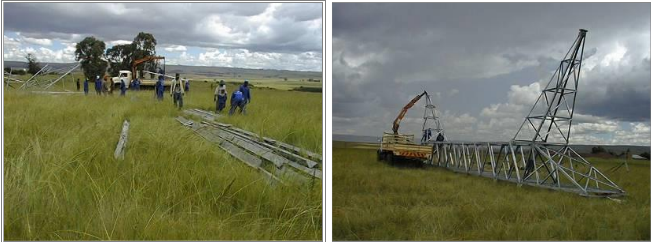
Figure 29: Delivery of steel (top) and assembly of tower (bottom)
