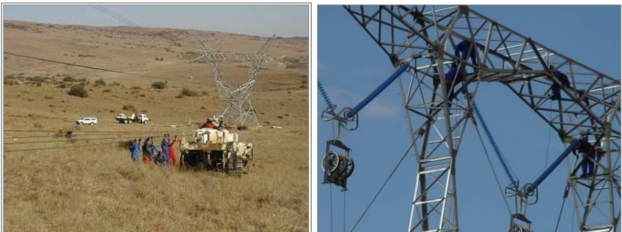
Figure 32: Stringing with pilot tractor (top) and pulleys (bottom)
