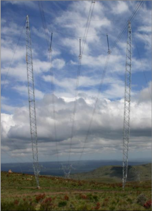
Figure 18: Tower Type 438 A - Cross Rope Suspension tower
