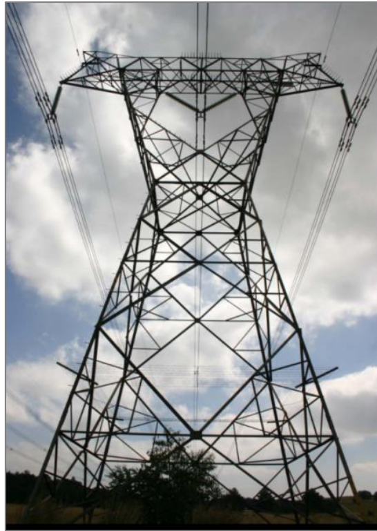
Figure 20: Tower Type 433A = Self Supporting Suspension tower
