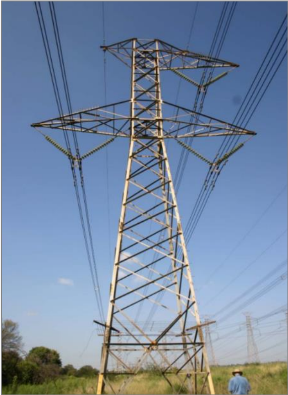
Figure 19: Tower Type 424 A - Self Supporting Suspension tower
