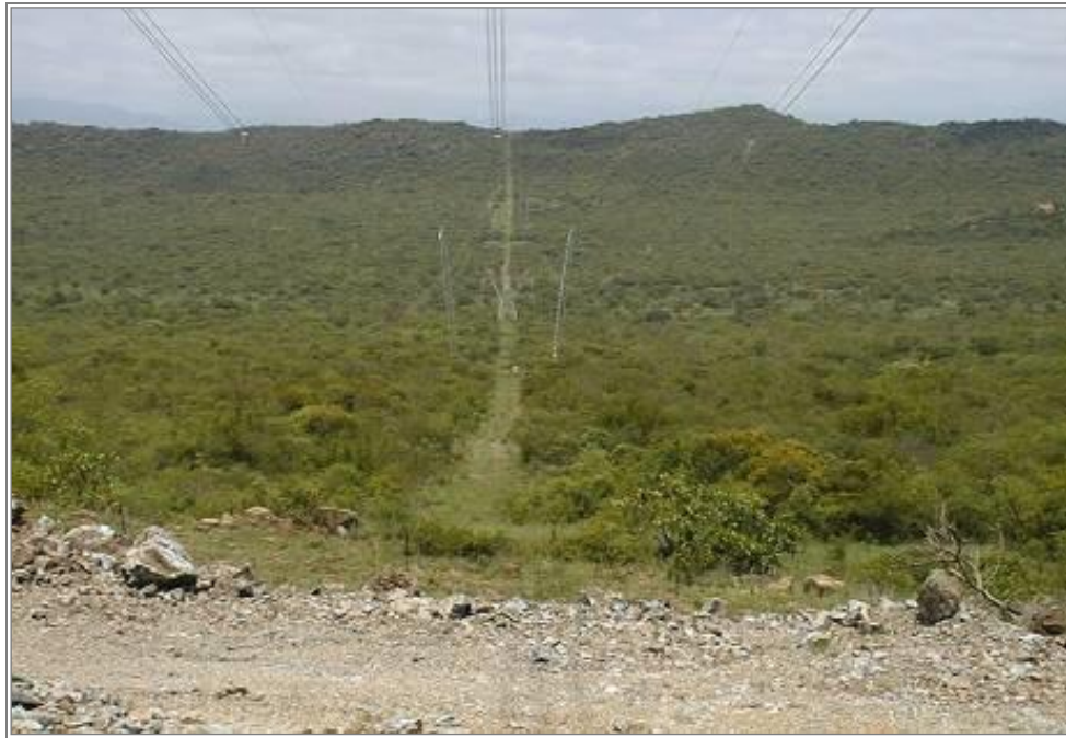
Figure 23: Vegetation clearance for stringing
