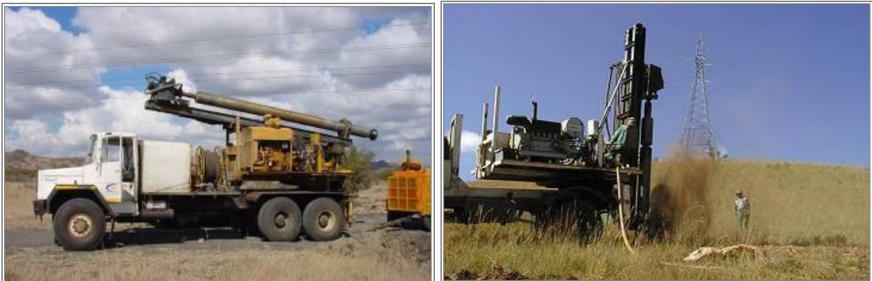
Figure 27: Drilling rig and generator (top) and excavation activities (bottom)
