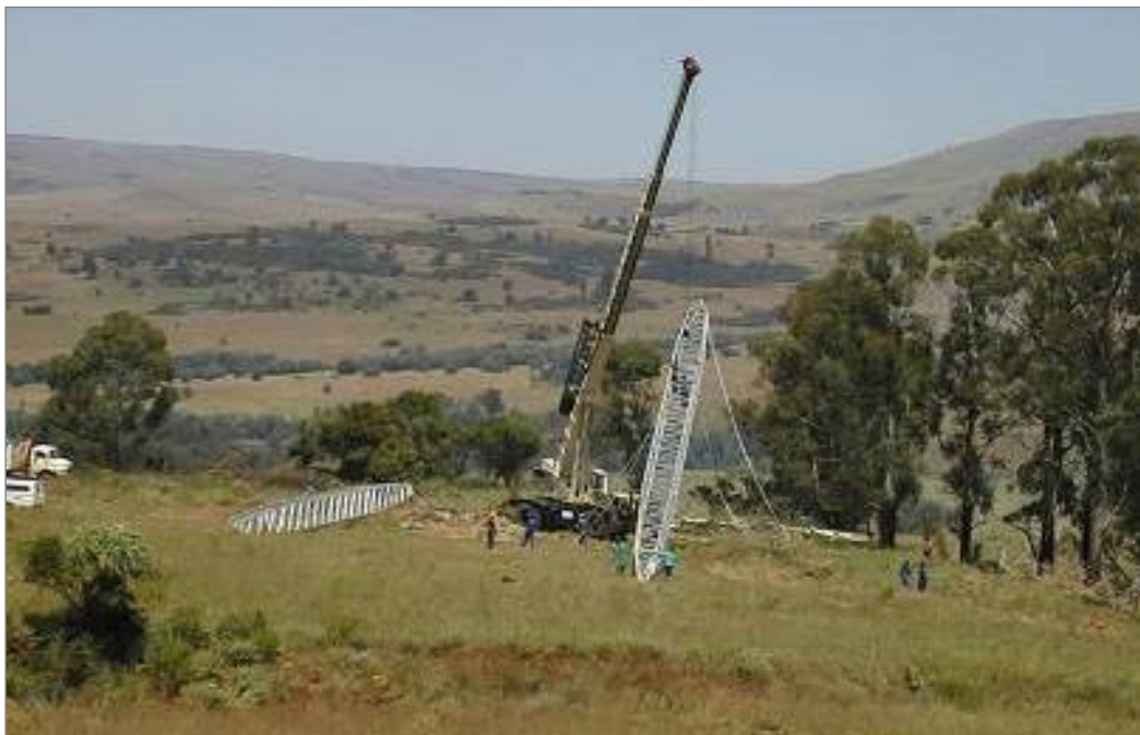
Figure 30: Erection of towers
