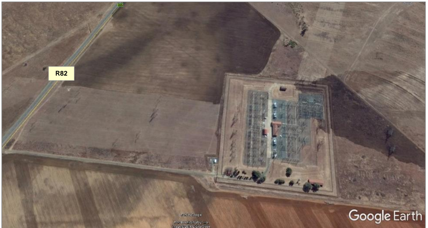
Figure 7: Makalu substation (Google Earth image)
