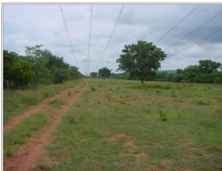
Figure 33: Example of an access road used for maintenance
