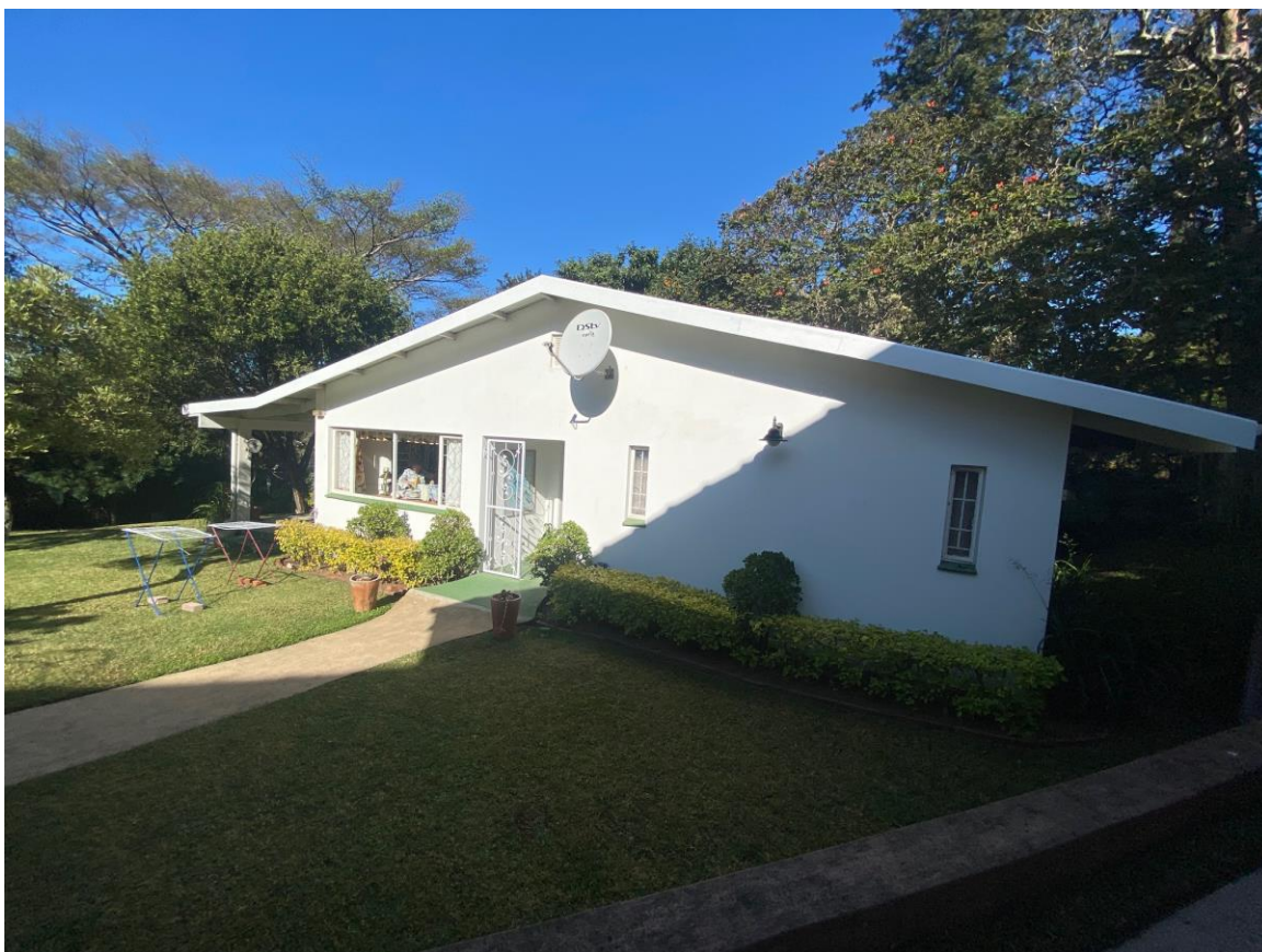
17. IMAGE N – NORTH WEST ELEVATION – EXG. SECOND DWELLING
