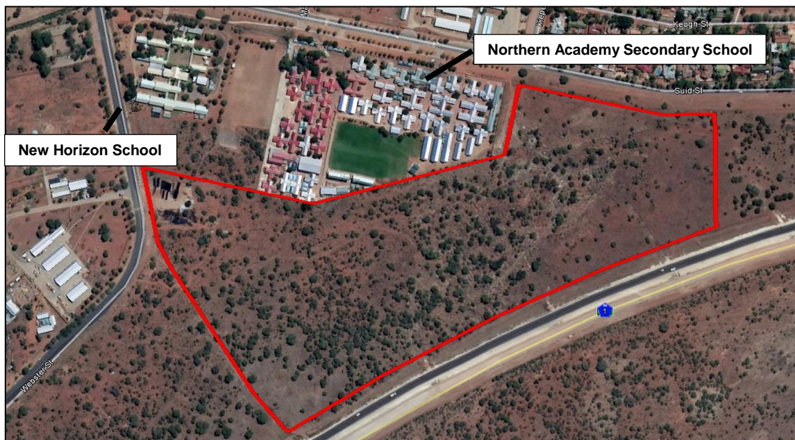
Figure 39: Existing infrastructure surrounding proposed site
