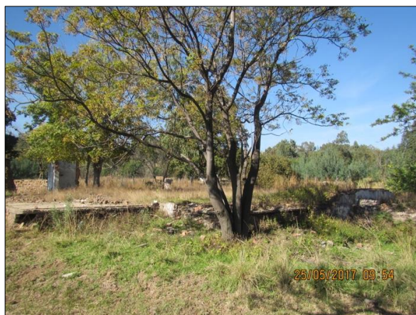
Figure 18: View of DUV001, showing the foundation of one of the buildings
