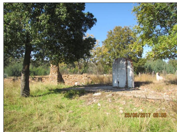
Figure 19: DUV001, showing boundary wall and remains of structure outside the wall
