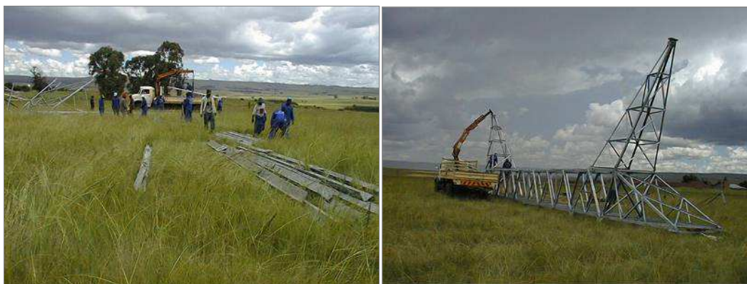
Figure 23: Delivery of steel (left) and assembly of tower (right)
