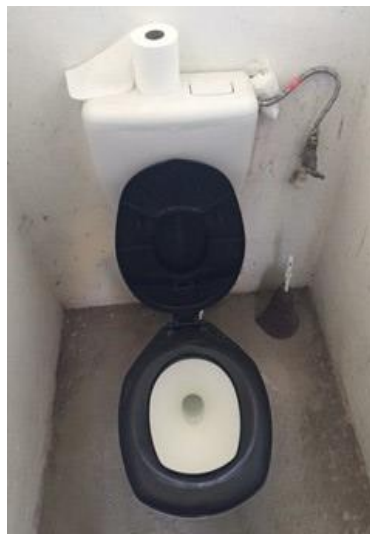
Figure 5: In House LVFT with Cistern
