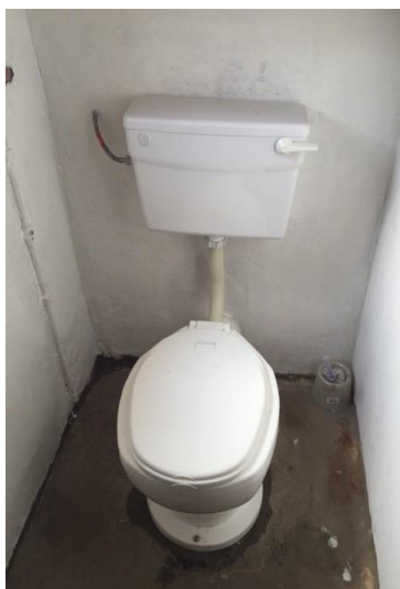
Figure 4: Outside LVFT With Cistern
