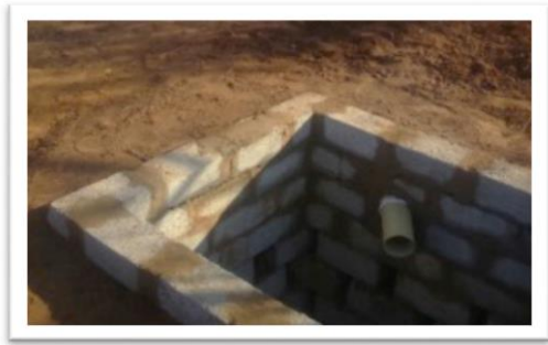
Figure 7: Leach Pit Construction
