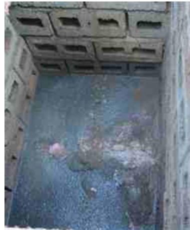
Figure 8: Active Leach Pit Contents
