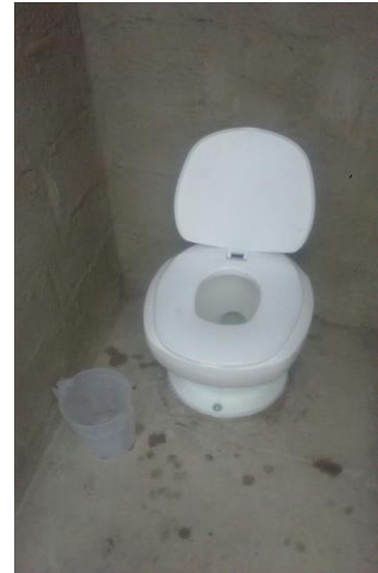
Figure 6: Pour-Flush LVFT
