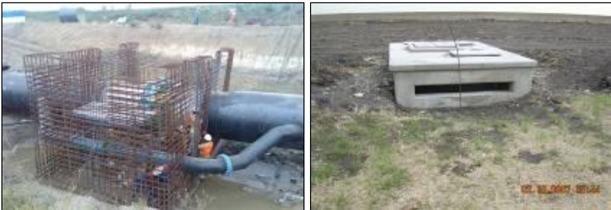
Figure 19: Typical examples of chambers (left - during construction; right – completed)
