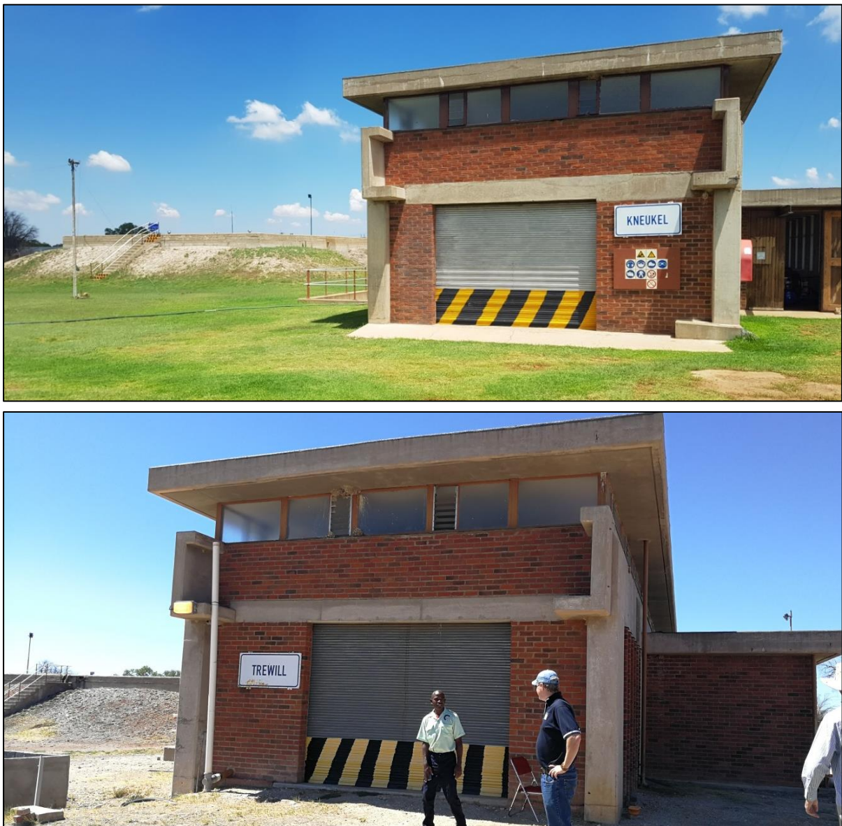
Figure 10: Kneukel (top) and Trewill (bottom) Pump Stations and Sumps
