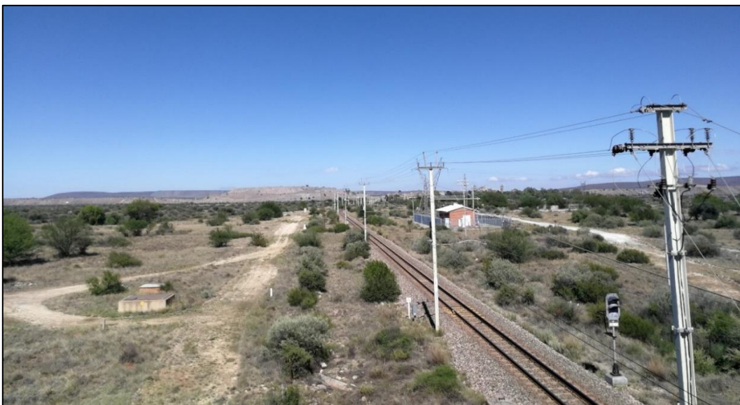
Figure 58: View along railway line (existing pipeline on left-hand side)
