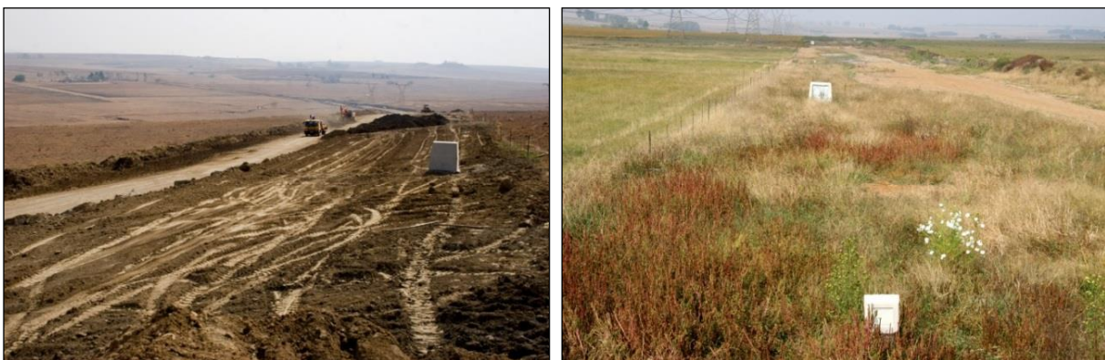
Figure 20: Typical views of reinstated (left) and rehabilitated (right) pipeline routes
