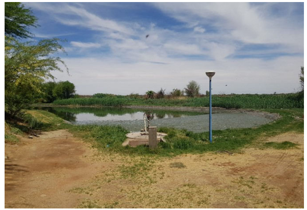
Figure 6: Emergency pond at K-WWTW
