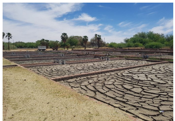
Figure 7: Sludge drying beds at K-WWTW
