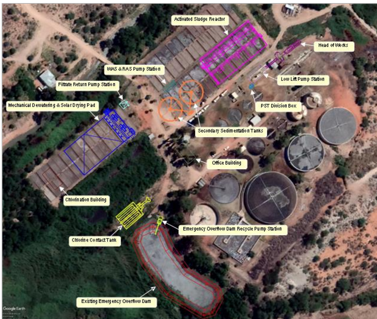
Figure C: K-WWTW upgrade and expansion works (Google Earth image)
