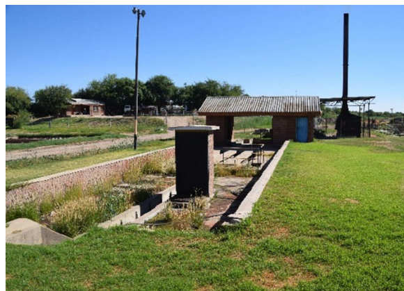
Figure 5: Obsolete “old” inlet works
