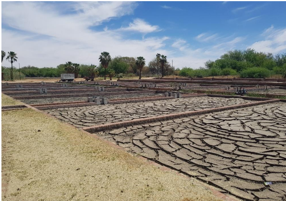
Figure 5: Existing sludge drying beds at K-WWTW
