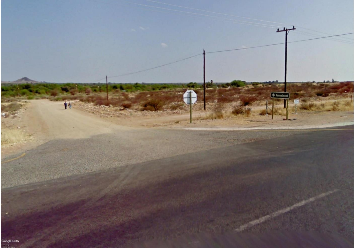
Figure 14: Access road to the K-WWTW from the N14 (Google Earth image)
