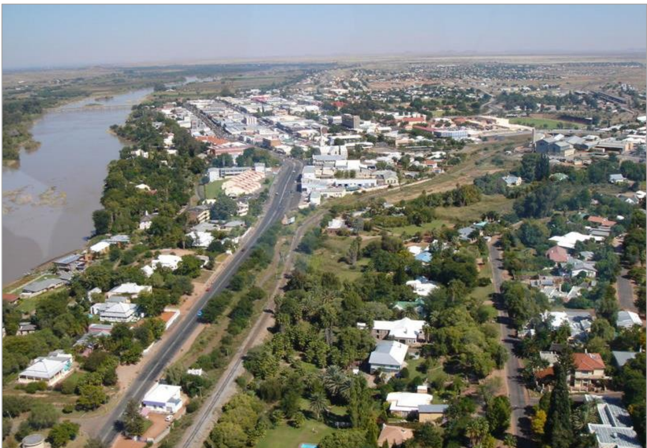
Figure 28: Aerial view of Upington's central business district ( https://commons.wikimedia.org/wiki/File:Upington.jpg )
