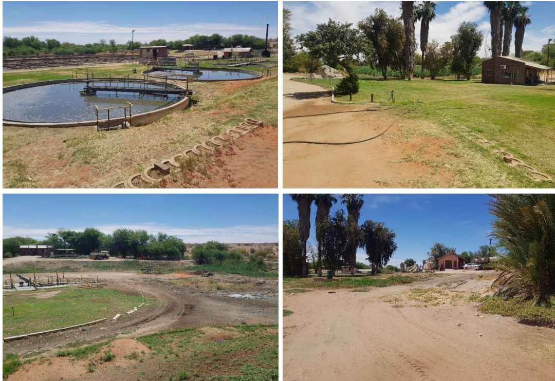
Figure 25: Photographs of the K-WWTW showing the degraded state of the vegetation
