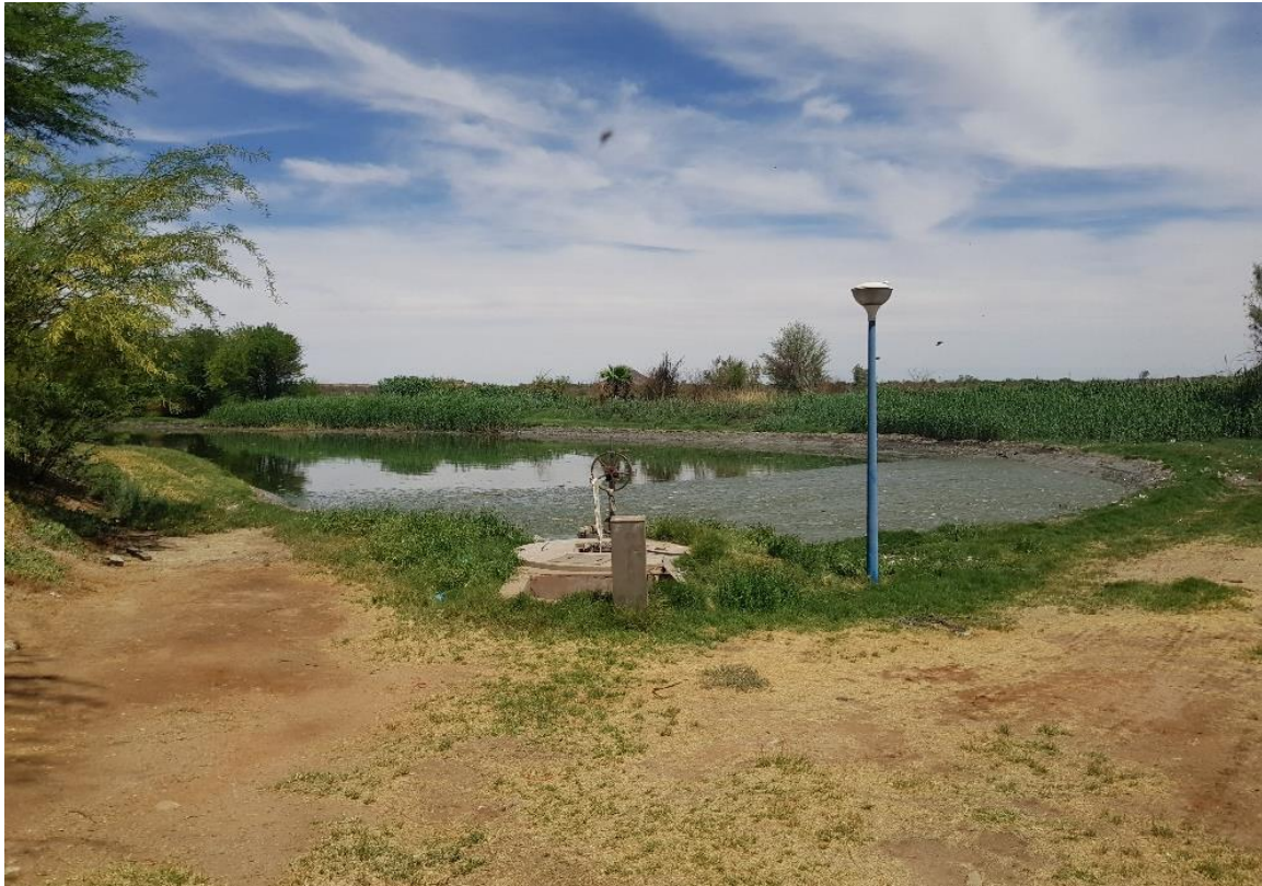
Figure 11: Emergency pond at K-WWTW
