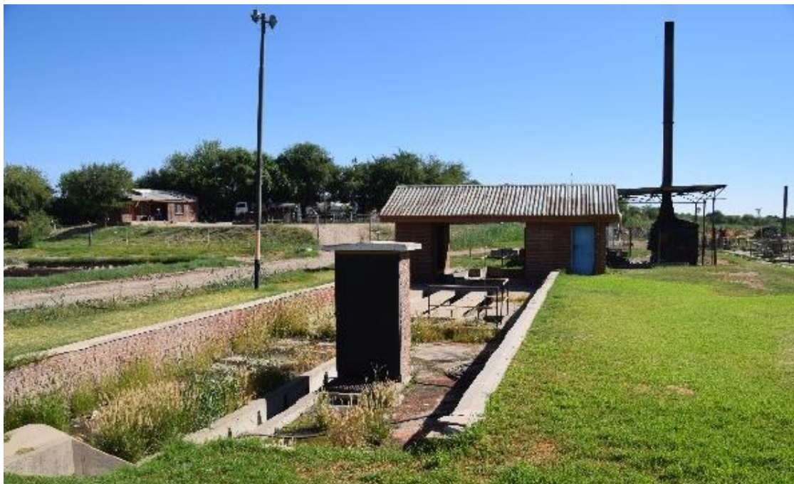
Figure 8: Obsolete “old” inlet works
