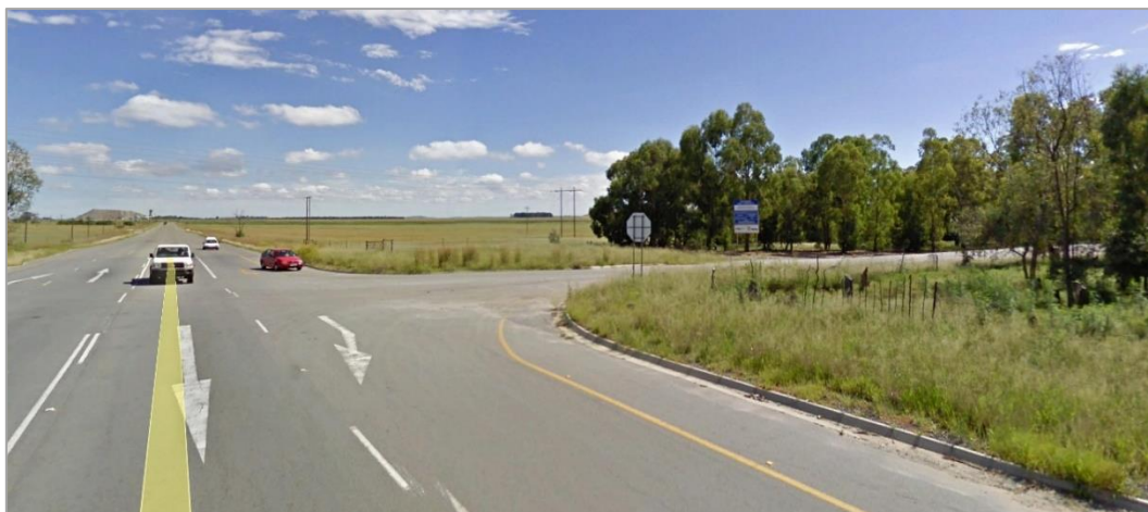
Figure 55: Northern view along the R33 (main access to site located to the left) (Google Earth image)
