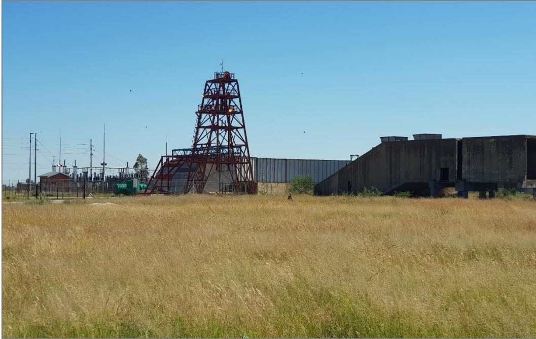
Figure 47: Vent shaft and sub-station – Phase 1 Site
