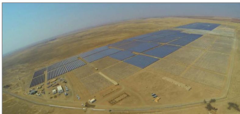
Figure 11: A Solar PV Plant under construction in SA
