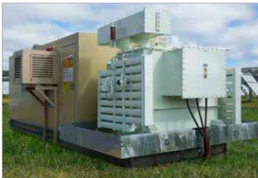
Figure 14: Example of Medium Voltage Transformer and Distribution Box (Photo from Actom Brochure)
