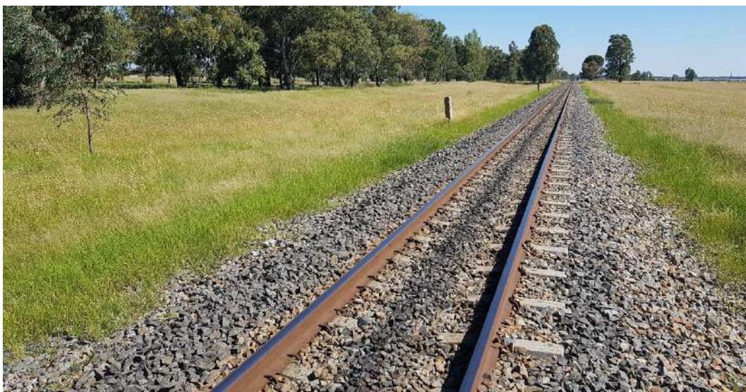
Figure 62: Southern view along the railway line (primary site located to the right)
