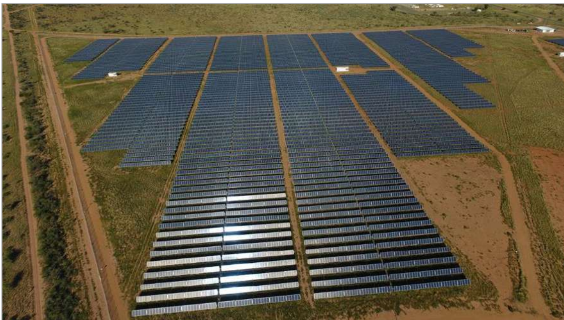
Figure 18: Example of Roads Between Trackers and Medium Voltage Substations (Photo from PIA Solar)
