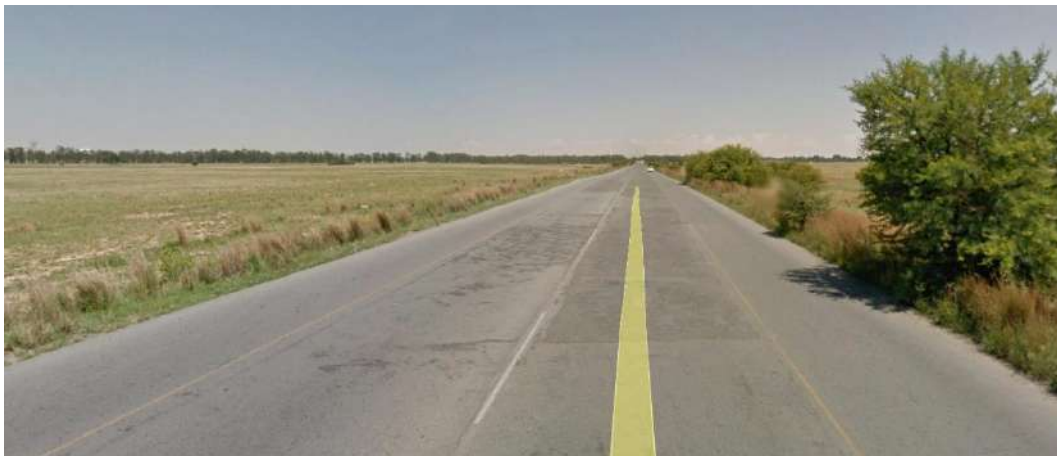
Figure 58: North-western view along the R70 (primary site located to the left) (Google Earth image)
