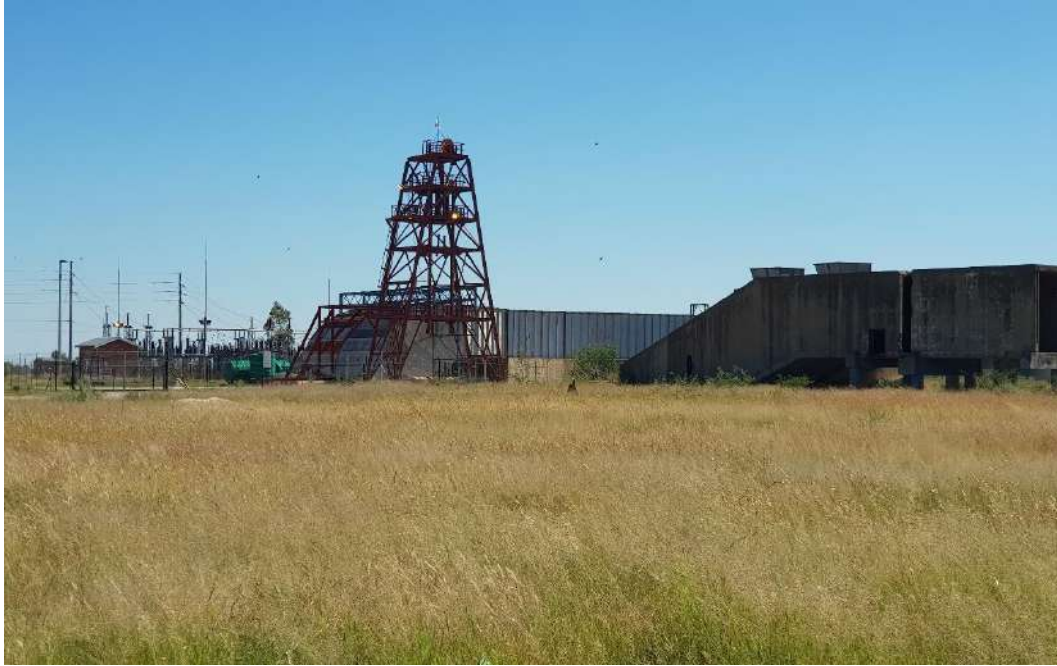
Figure 57: Vent shaft and sub-station – Phase 1 Site
