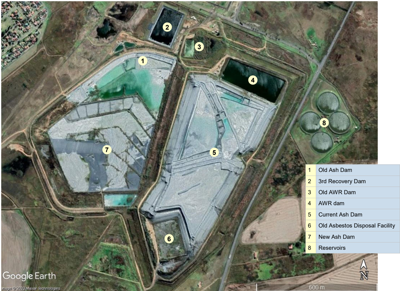
Figure 4: Ash dam area
