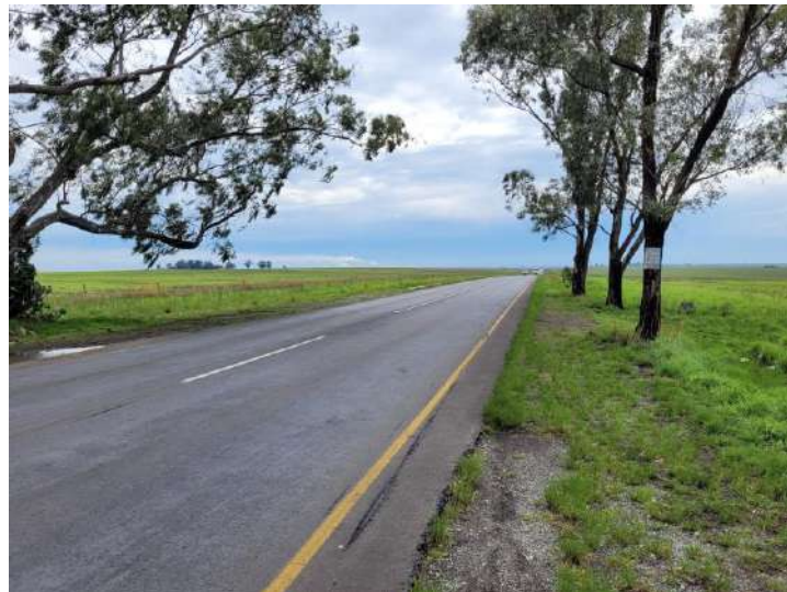
Figure 78: View along the R29 near the drill site
