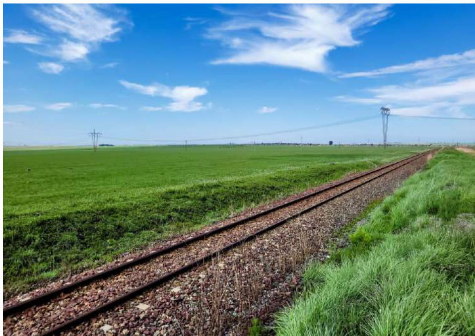
Figure 14: Railway line along the southern boundary of the drill site
