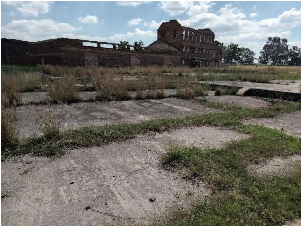
Figure 85: View of the foundations with the remains of the mill buildings in the background
