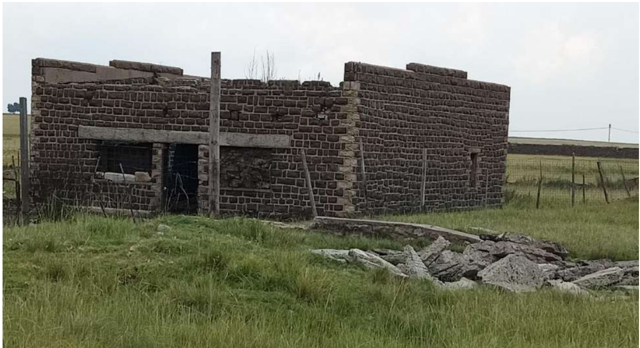
Figure 52: The building built with dolerite stone and sandstone details at the corners and windows, note the demolished material in the foreground
