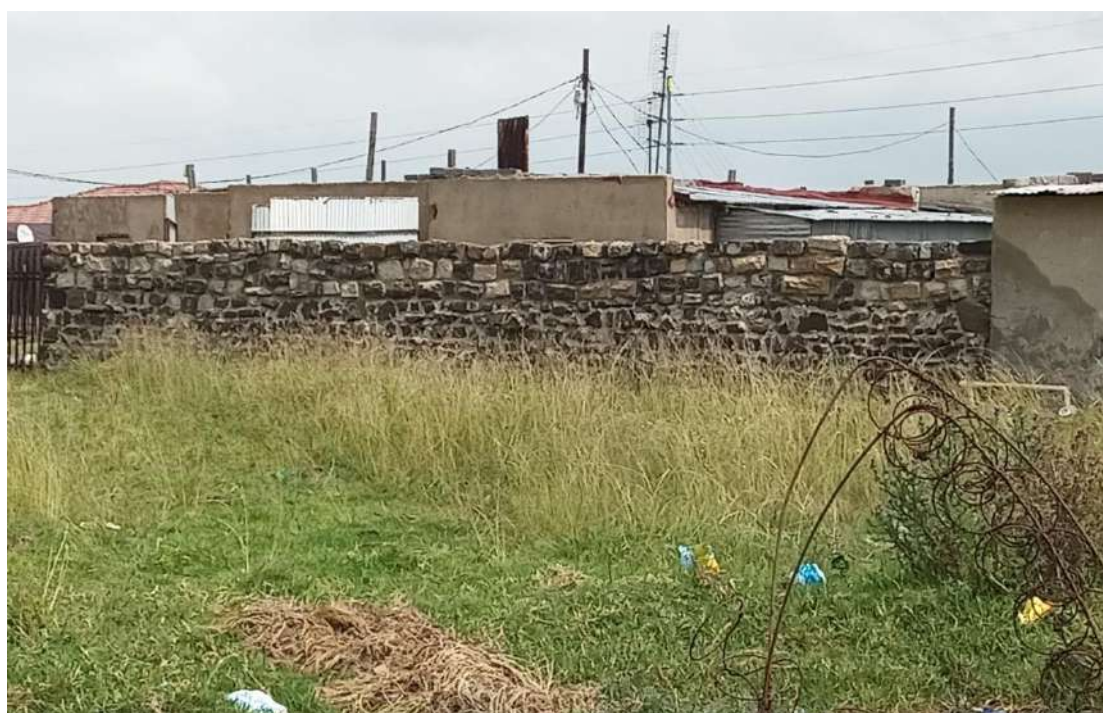
Figure 31: View of the old stone wall enclosing modern/recent structures
