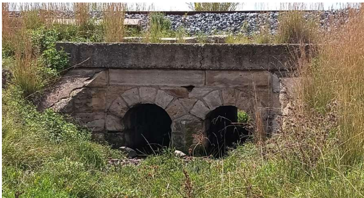
Figure 76: View of the double-arched railway culvert at CCUS-19
