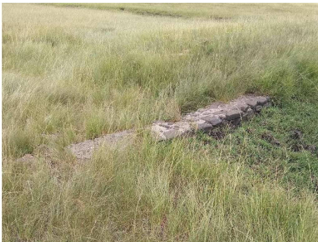
Figure 44: View of the stone dam wall/weir structure
