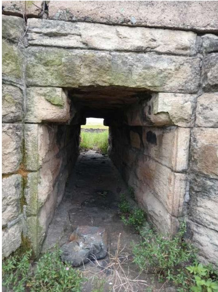
Figure 28: View of the stone culvert under the railway line at CCUS-03. This seems to be an example of a flat lintel or box culvert.
