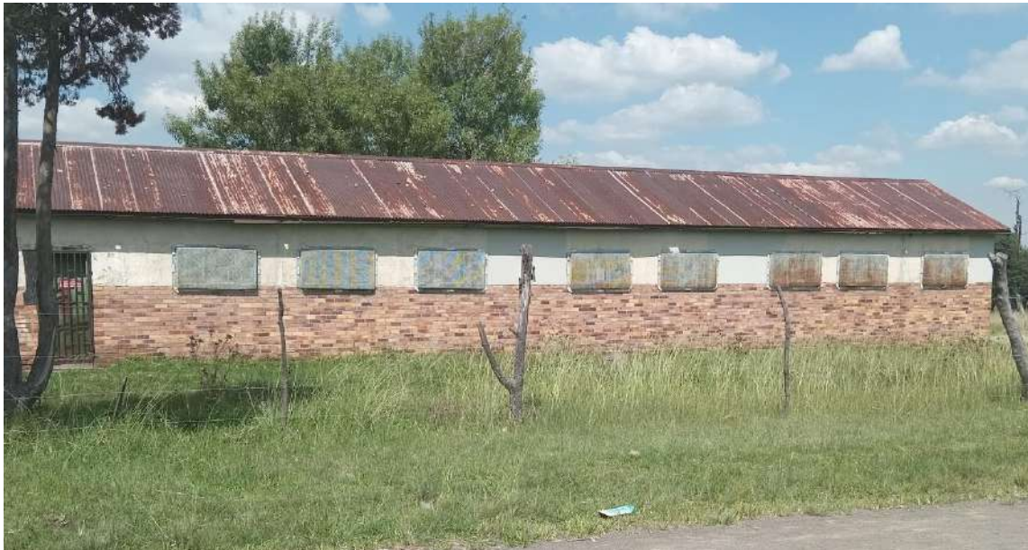
Figure 94: View of the third building
