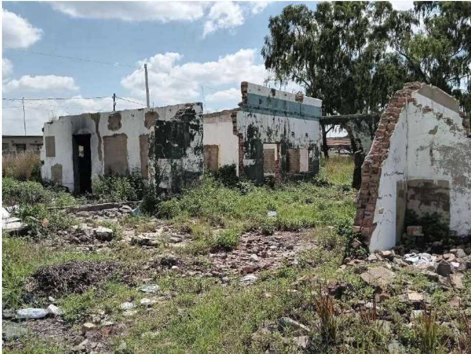
Figure 78: View of the ruined structures at CCUS-21
