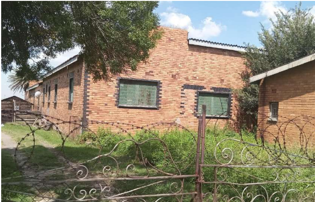
Figure 92: View of one of the three other buildings at CCUS-27, showing the blue/purple brick detailing
