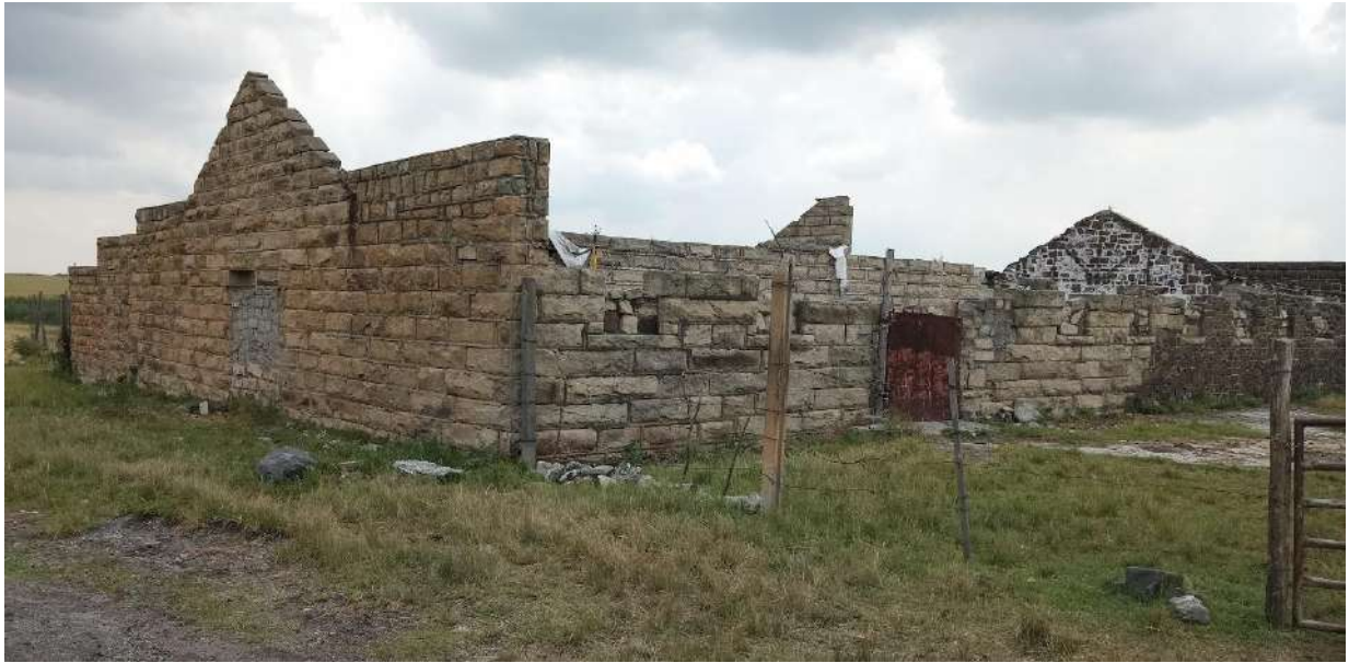
Figure 53: View of the larger building, one section of which is constructed sandstone
