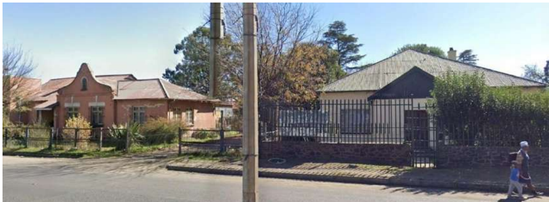
Figure 13: View of two historical houses on the north side of the Leandra Main road/R29 (Google earth Streetview)
