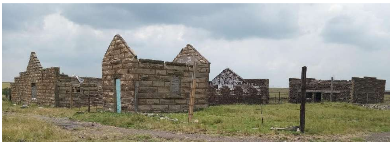
Figure 50: General View of the three buildings at CCUS-13
