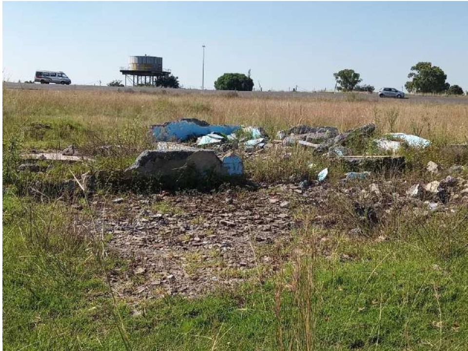
Figure 95: View of demolished remains of building at CCUS-29
