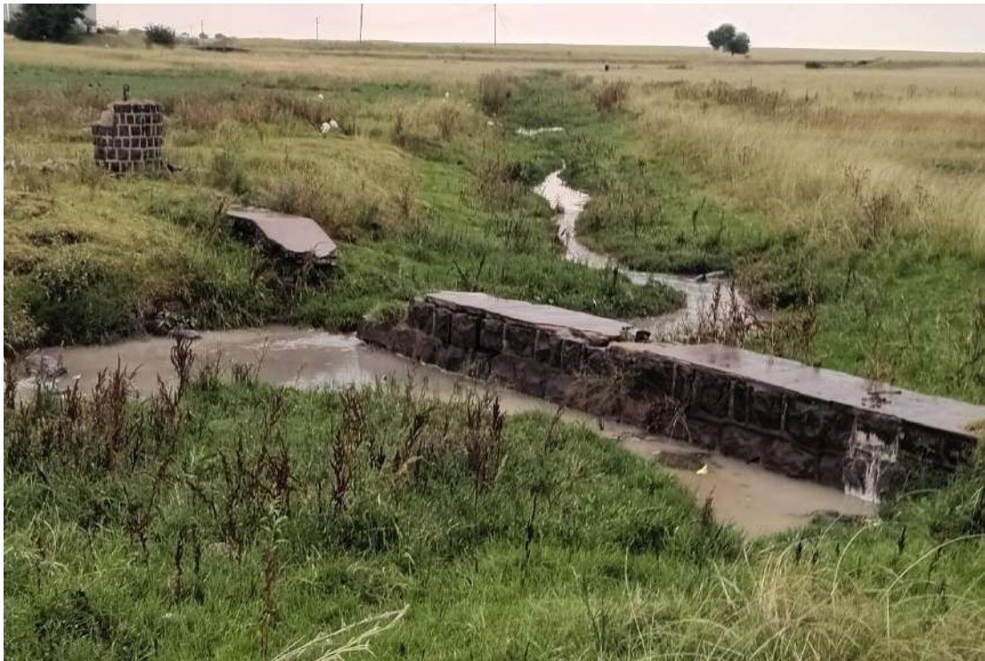
Figure 62: View of the remains of the historical stone bridge at CCUS-15
