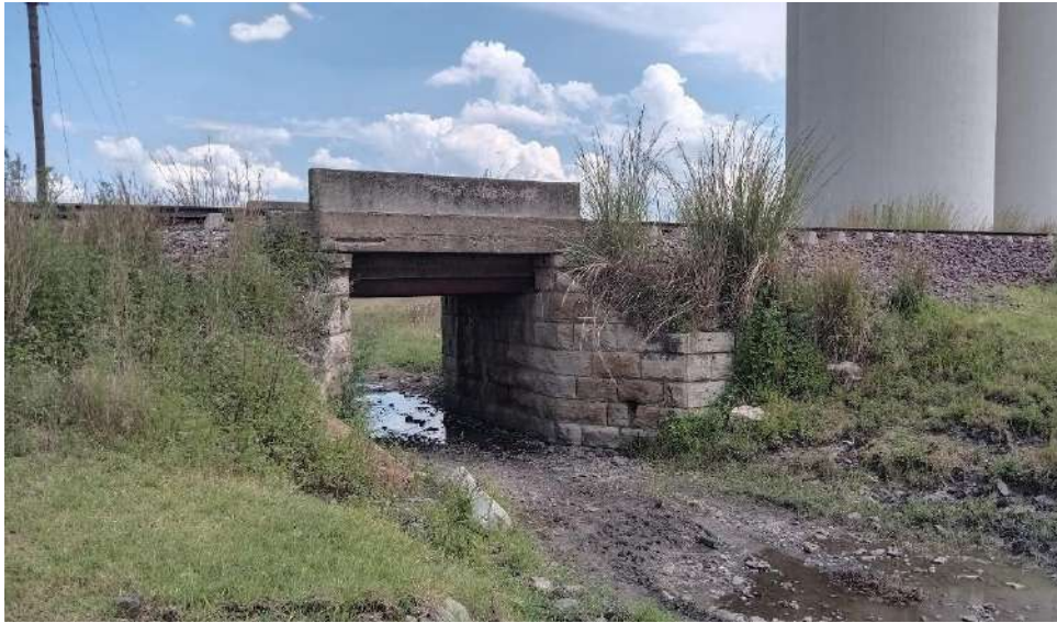
Figure 109: View of historical stone culvert under railway line at CCUS-33
