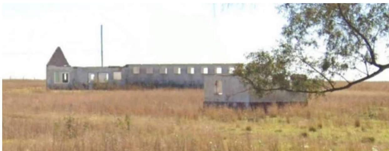
Figure 72: View of the two old and dilapidated buildings at CCUS-17
