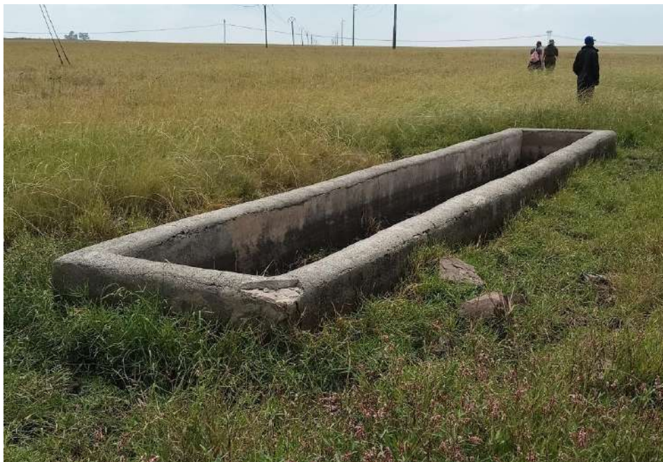
Figure 37: View of large trough, covered in cement
