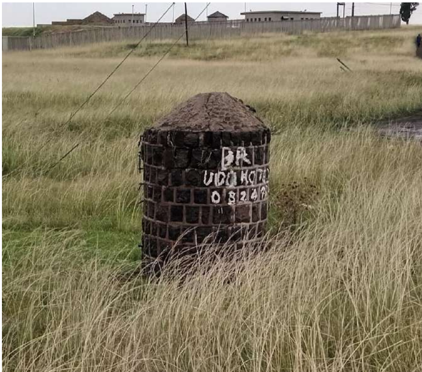
Figure 63: View of the circular pillar associated with the bridge remains
