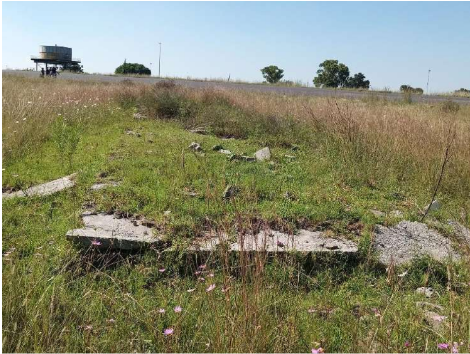
Figure 97: View of one of the foundation remains at CCUS-29
