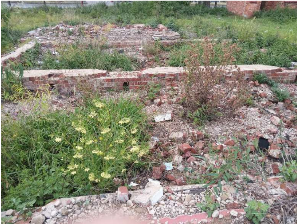
Figure 64: View of the foundation remains of one house built from red brick at CCUS-16
