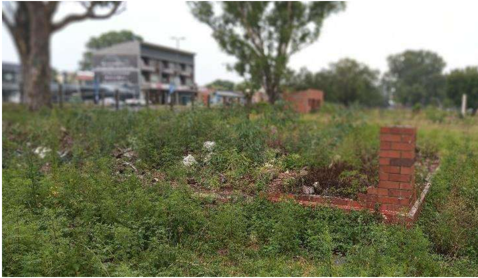
Figure 68: View of one of the foundations with piece of wall in red brick
