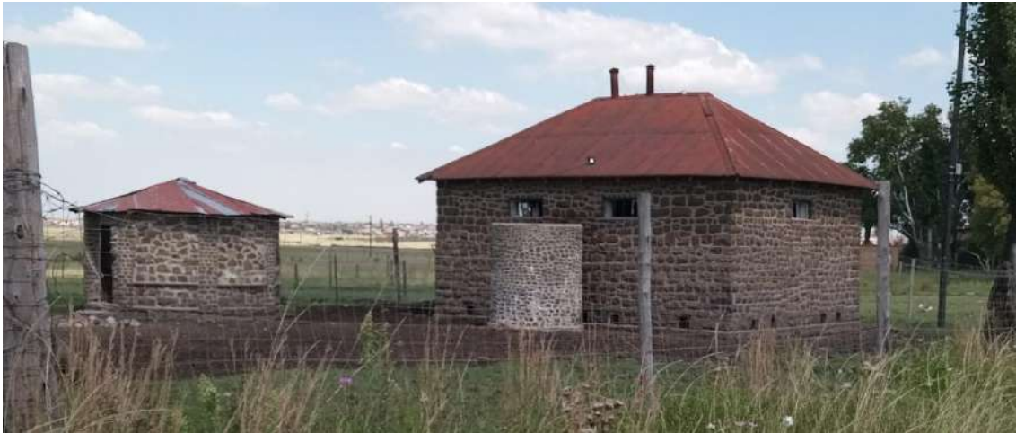
Figure 88: View of the two stone buildings at CCUS-26, note the circular feature at the side
