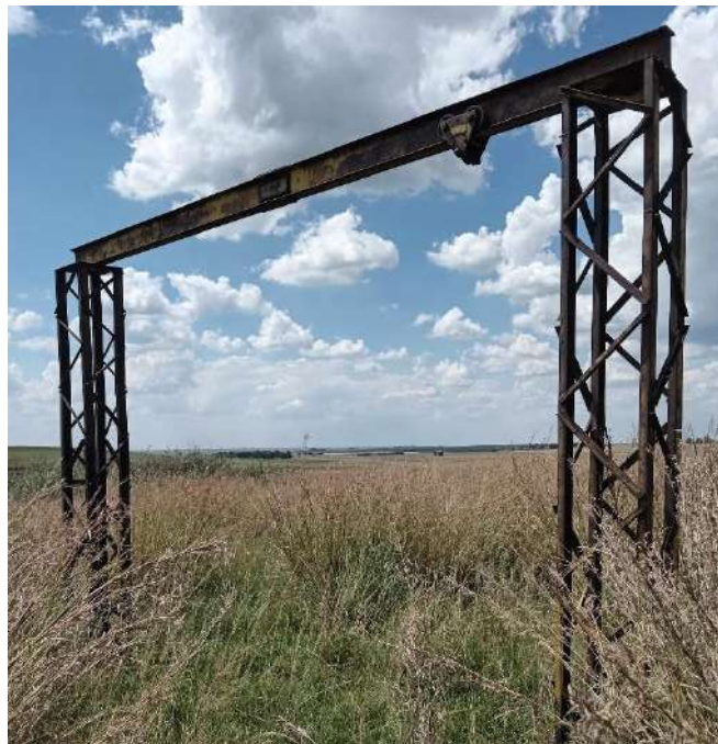
Figure 108: View of metal structure
