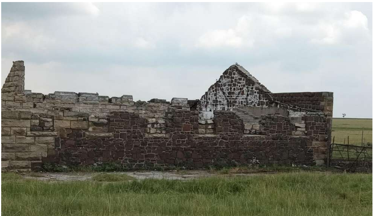
Figure 54: View of the other section of the larger building, which is partially constructed of dolerite
