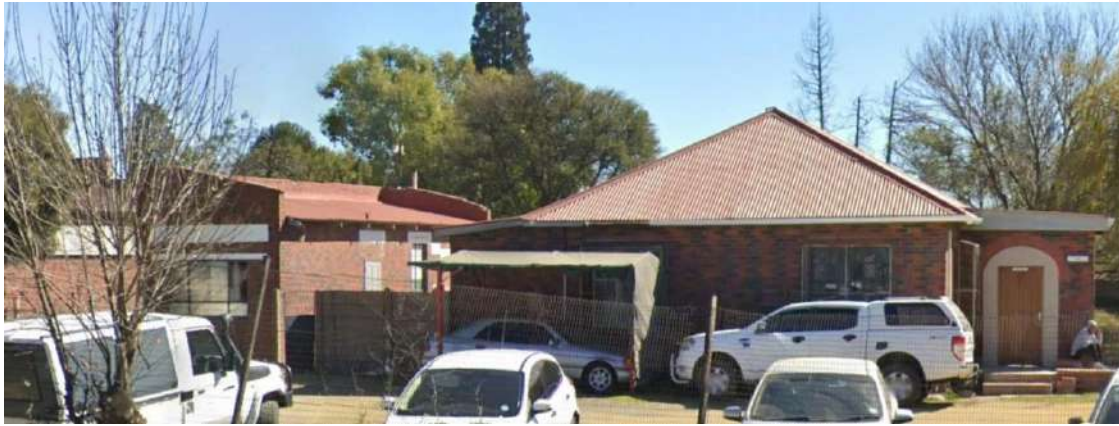
Figure 15: View of historical police station building on north side of Leandra Main Road/R29 (R29 (Google earth Streetview))
