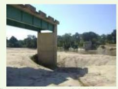
Figure 2 | Flood damage to existing bridge
