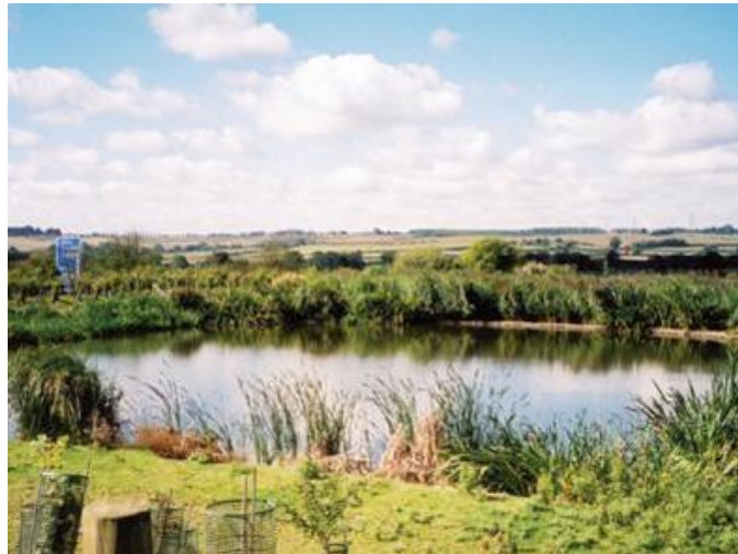
Figure 10.11: Typical stormwater attenuation pond (Hatch, 2013)
