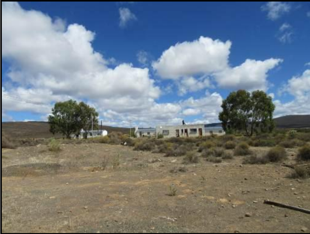
Photograph 1.8: Workers' houses on Fortuin
