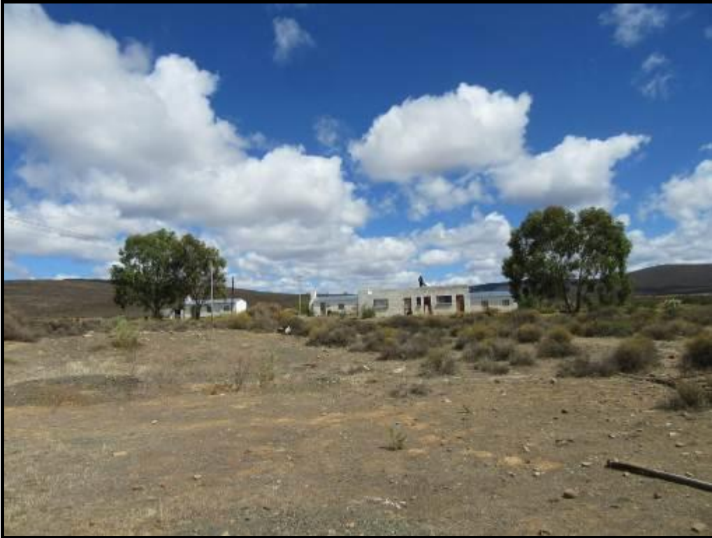
Photograph 1.8: Workers' houses on Fortuin
