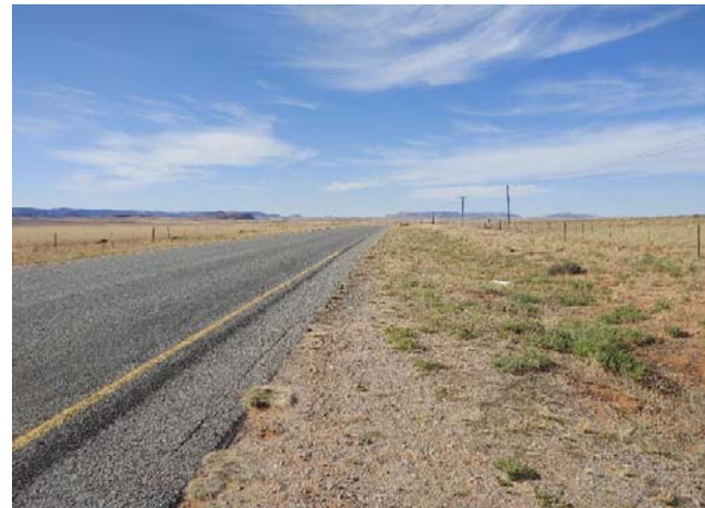
Photo 4: SSD to the East along the N14 from the Access (>500m)
