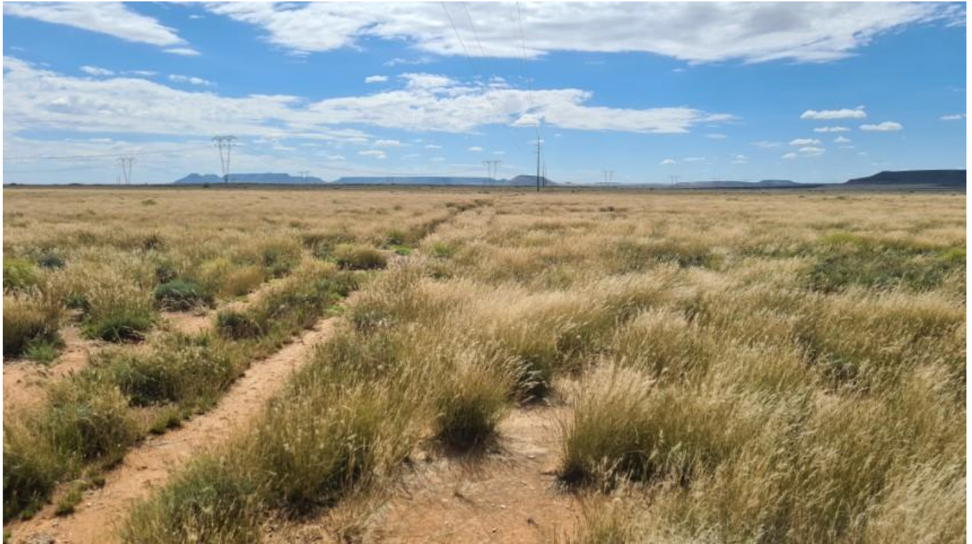
Figure 7: Existing HV powerlines within the study area
