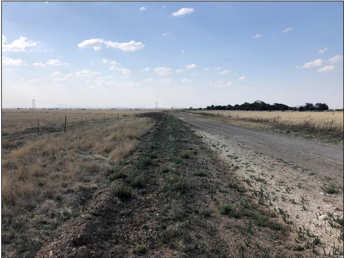
Figure 4.12: S322 gravel road adjacent site, taken towards the north
