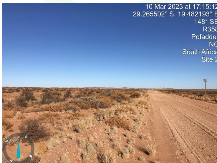
Figure 4.11: Wooden utility poles along the R358
