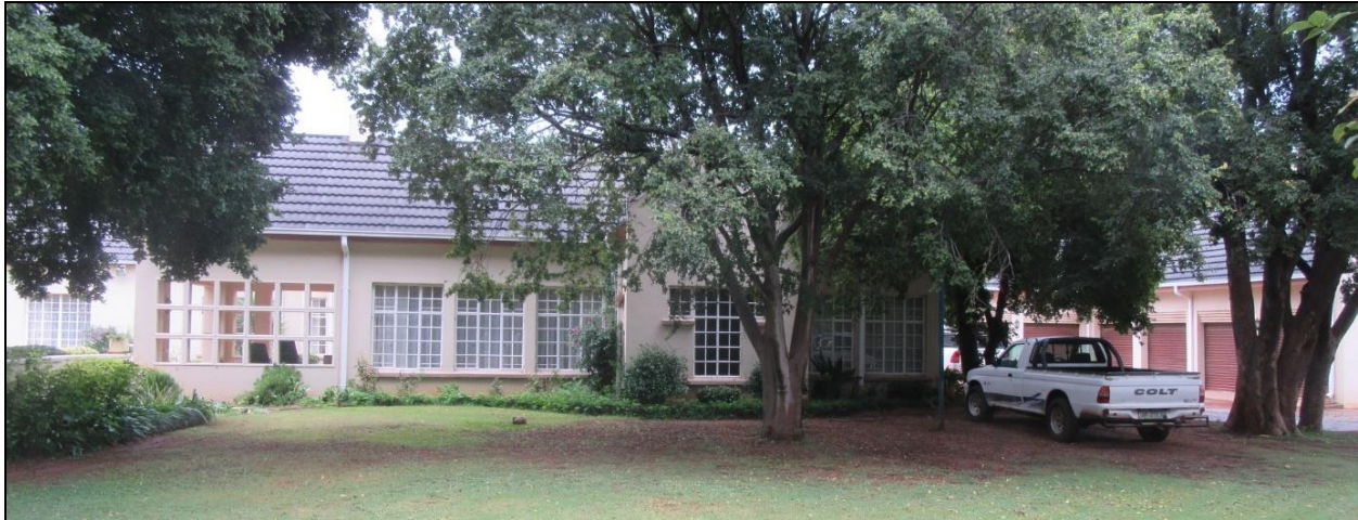
Photograph 3.11: Elandsfontein farmstead located just to the south of the Mahikeng road.
