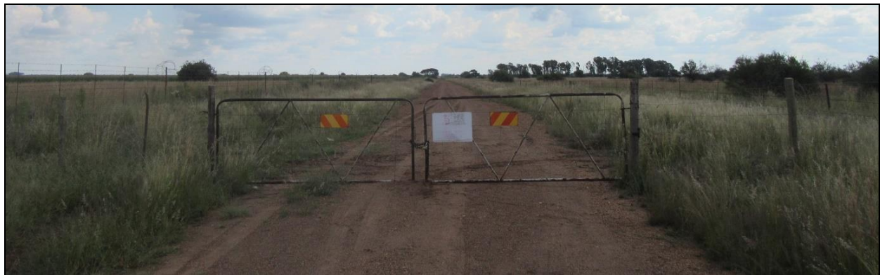
Photograph 3.11: Private access road to Sensako farm (site access road Alt 3) seen from across the R505 (Zeerust Road)
