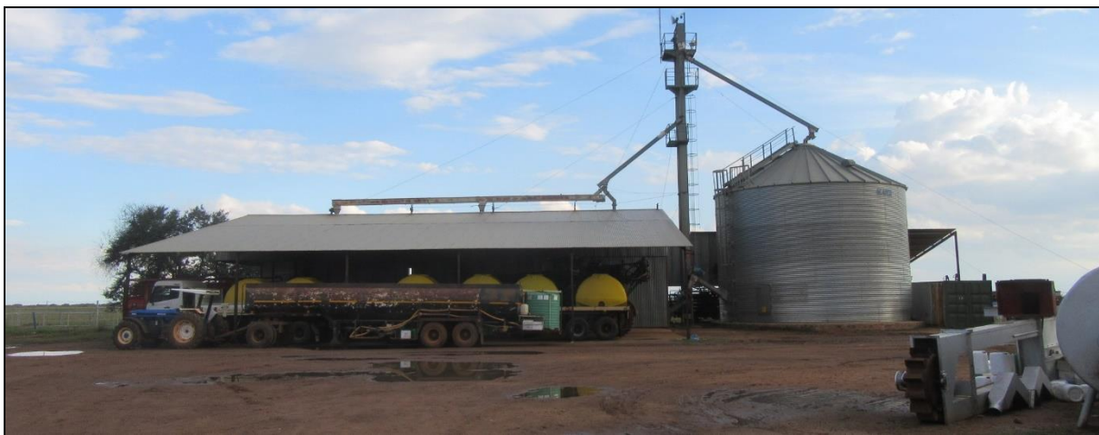
Photograph 3.13: Farm yard on Scherppunt
