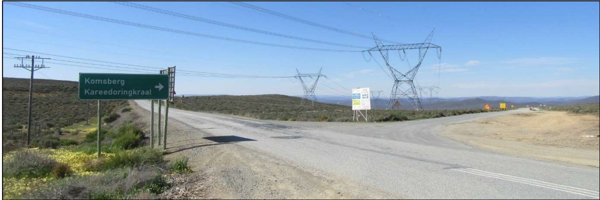
Photograph 3.1: Intersection of the R354 and Komsberg gravel road, viewed from the south. The power lines are 400 kV and 765 kV lines feeding into Komsberg substation.
