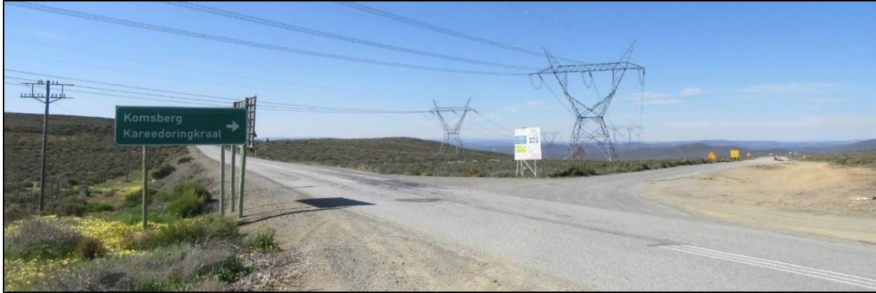
Photograph 3.1: Intersection of the R354 and Komsberg gravel road, viewed from the south. The power lines are 400 kV and 765 kV lines feeding into Komsberg substation.
