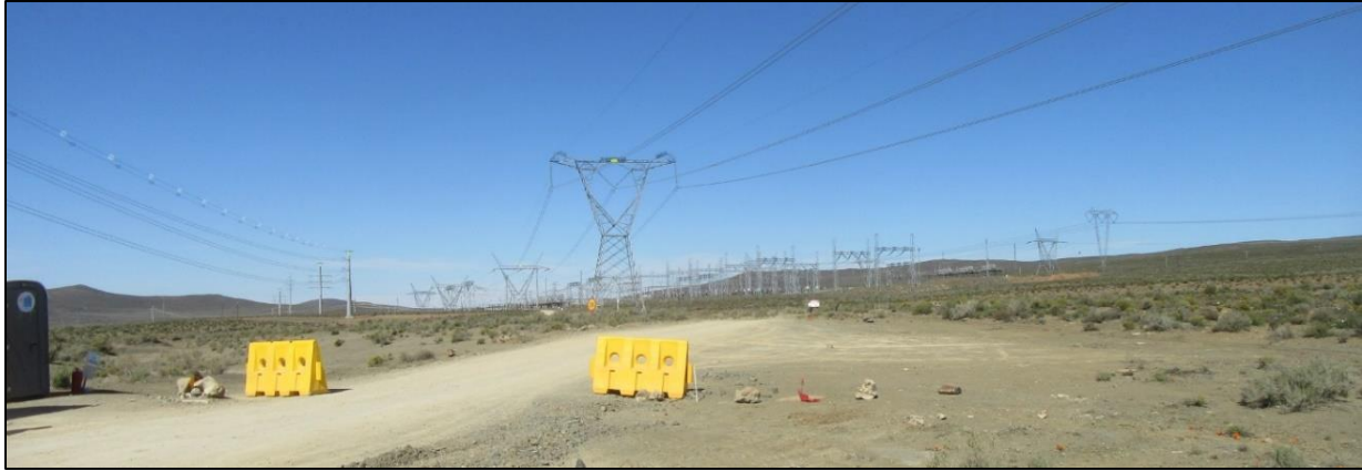
Photograph 3.2: Eskom's Komsberg substation, viewed from the entrance along the Komsberg Road.
