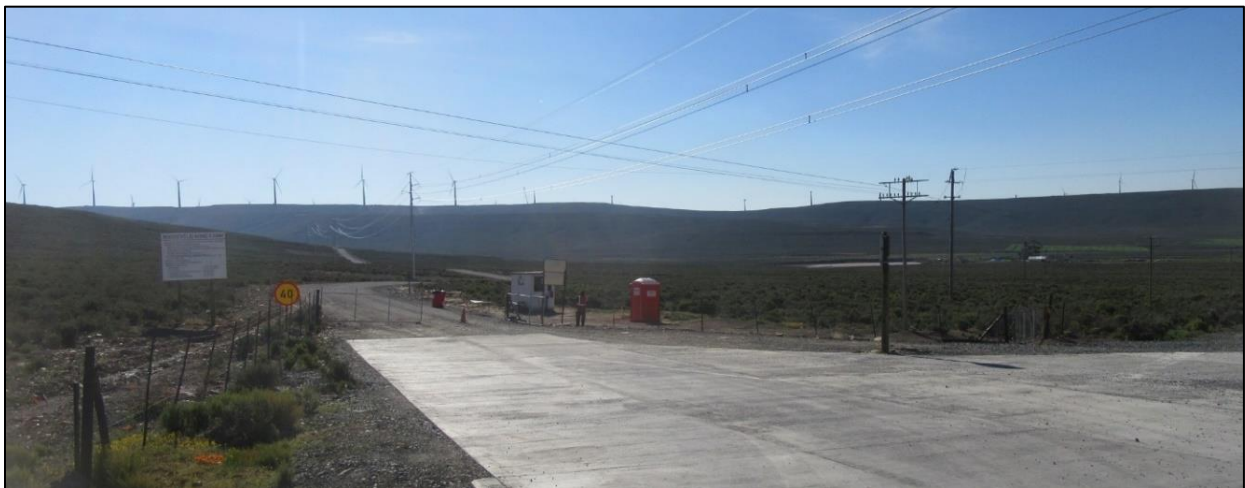
Photograph 3.3: Entrance to Roggeveld WEF off the R354 (Swartland farm).
