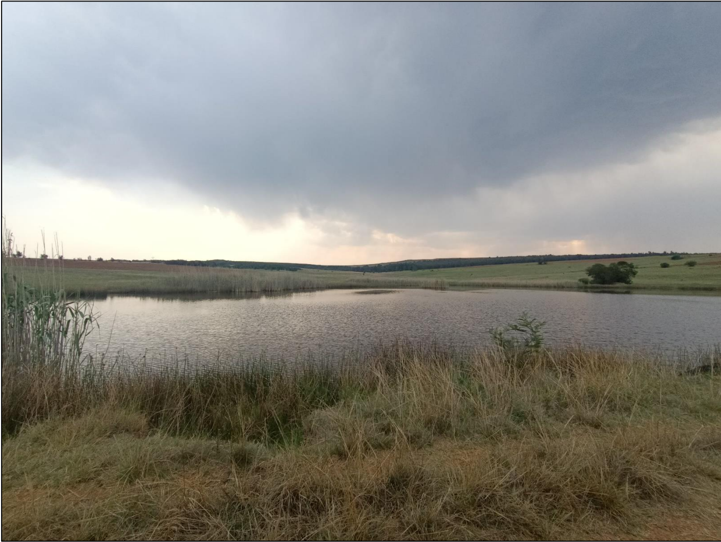
Example of a Focal Site dam on site
